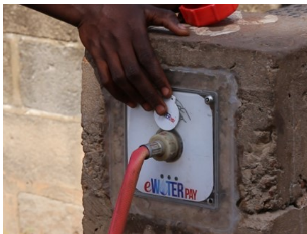
Figure 1. e-Tap and token in contact releasing water.
