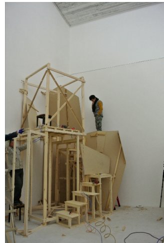
(b) The spiral staircase in construction
