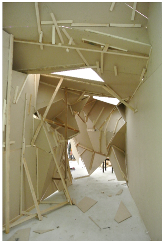
(a) View of the entrance in construction
