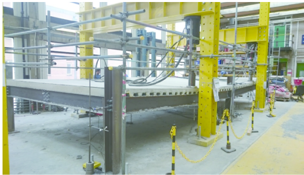
Fig. 22. Deflection of the edge beam due to missing support to the central column.
