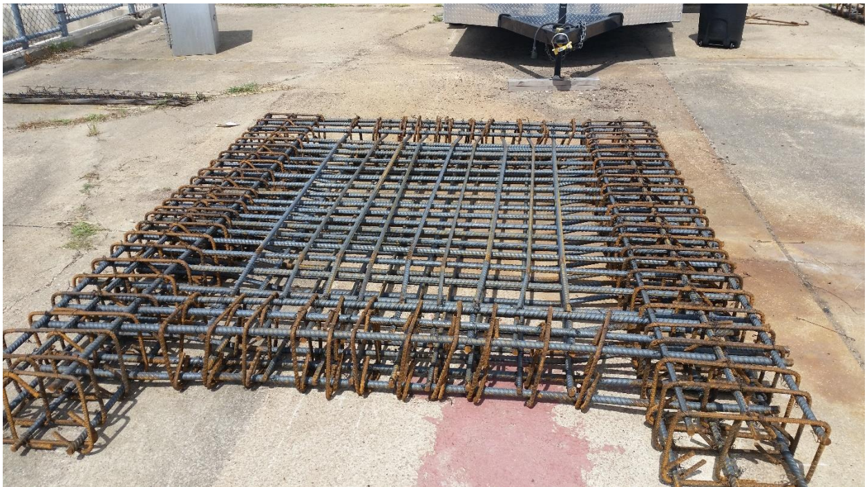
Figure 33 Specimen 1- Reinforcing Steel Assembled Cage
