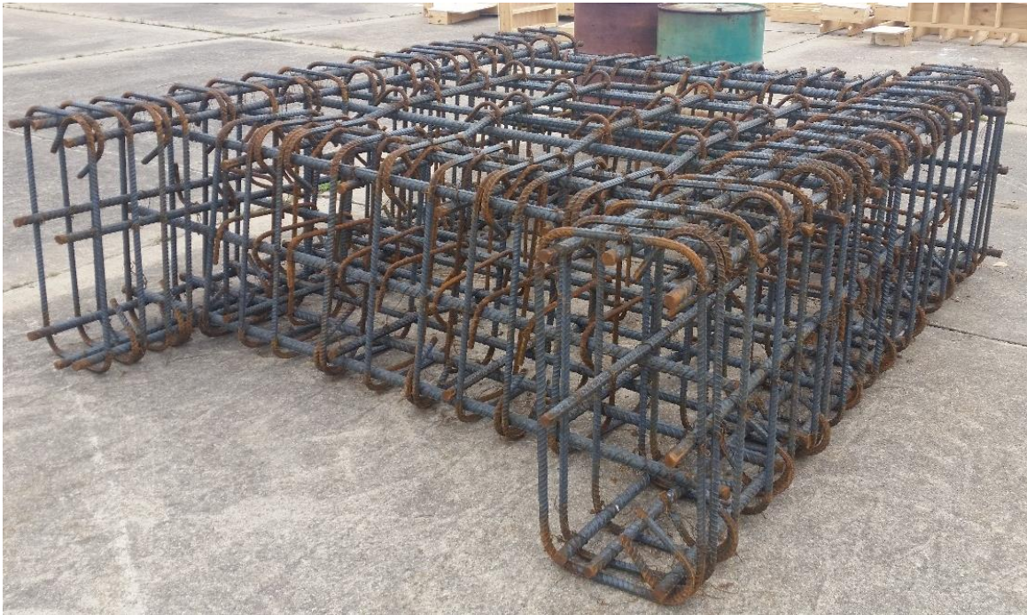
Figure 34 Specimen 2- Reinforcing Steel Assembled Cage
