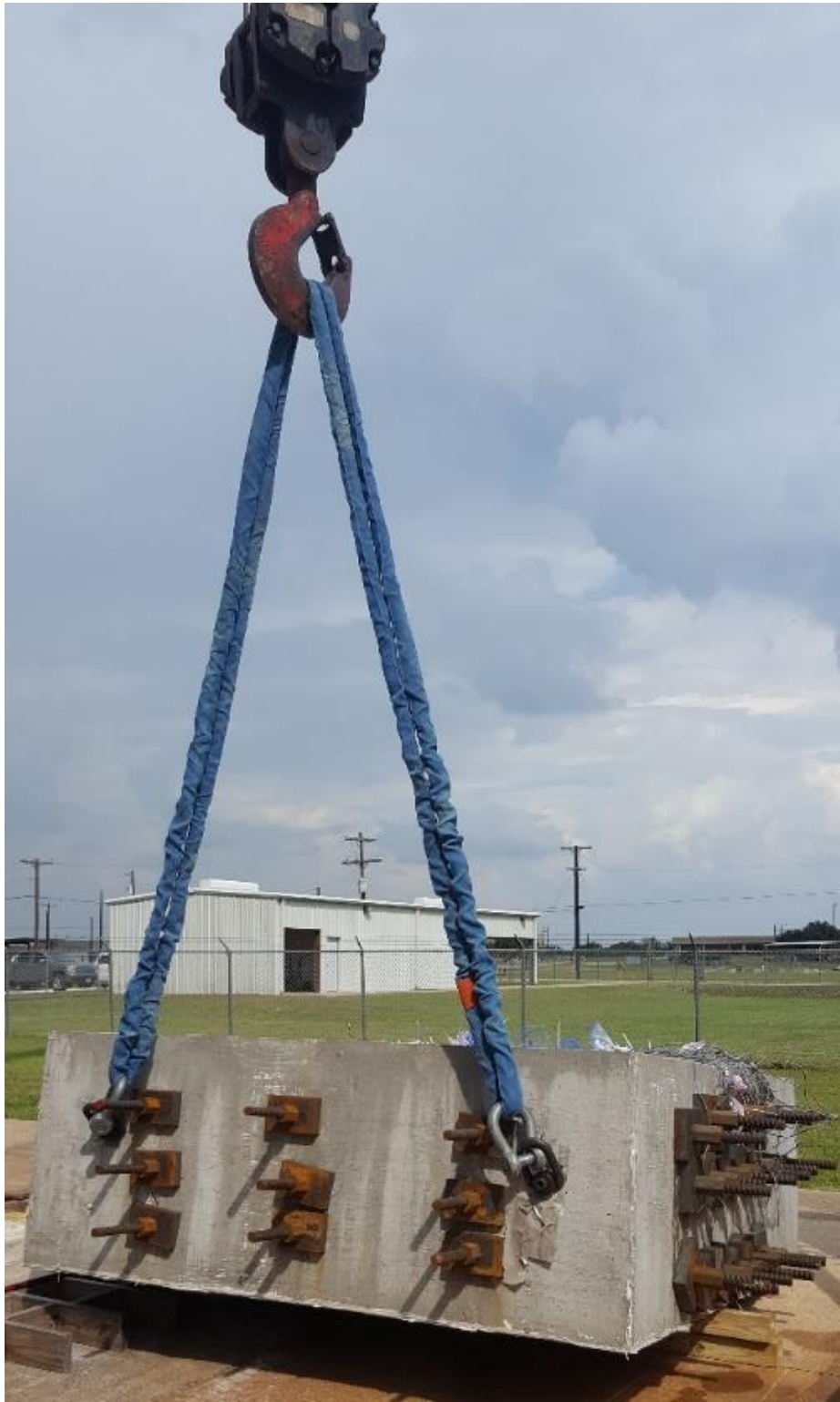
Figure 65 Specimen 2- Lifting Off Ground into Final Position
