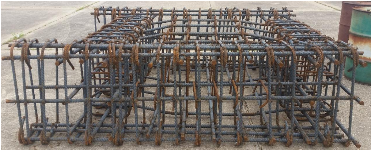
Figure 35 Specimen 2- Reinforcing Steel Assembled Cage
