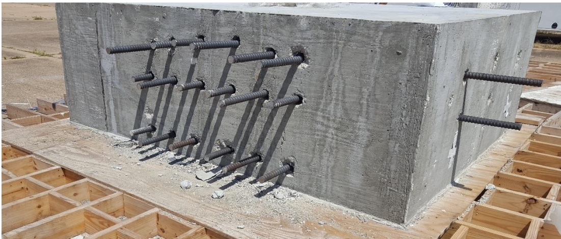
Figure 59 Specimen 2- Forms Stripped After Concrete Pour and Post-Tensioning Bars Installed
