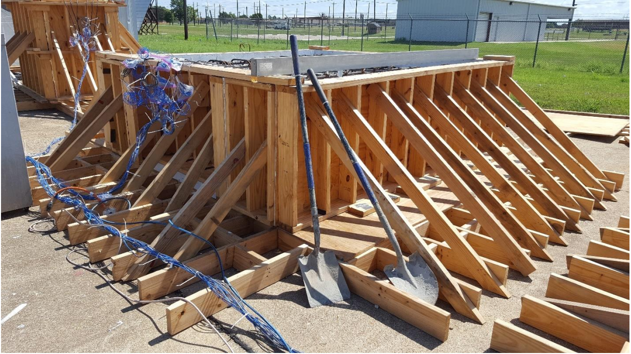
Figure 48 Specimen 2- Pre-Pour Set Up
