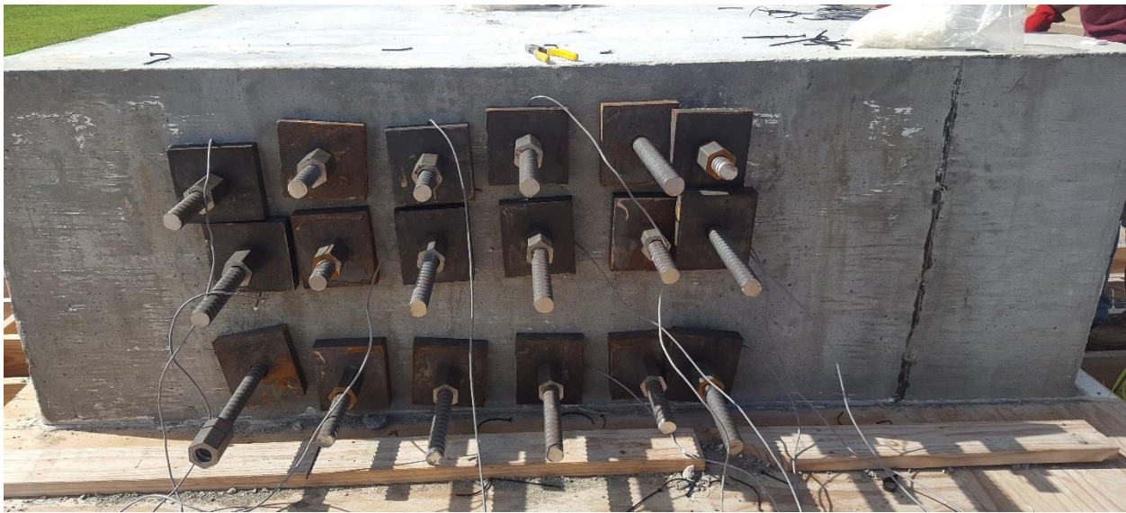
Figure 61 Specimen 2- Post-Tensioning Bars with Anchor Plates and Nuts, Side View
