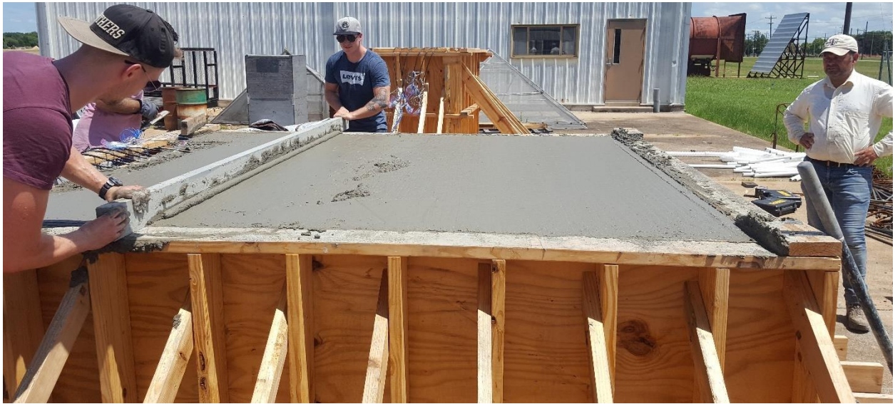
Figure 52 Specimen 2- Concrete Pour Finishing
