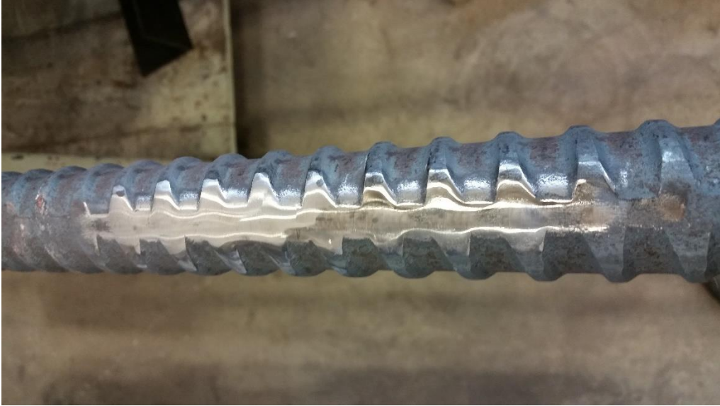
Figure 54 Post-Tensioning Bar After Grinding and Sanding
