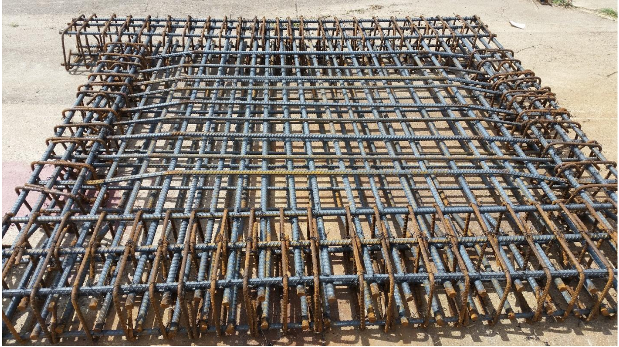
Figure 32 Specimen 1- Reinforcing Steel Assembled Cage
