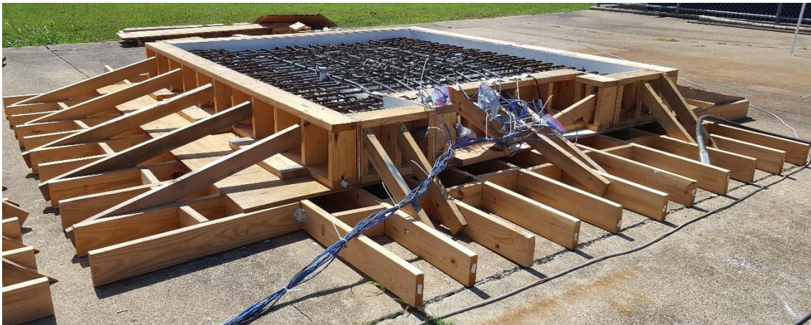
Figure 47 Specimen 1- Pre-Pour Set Up
