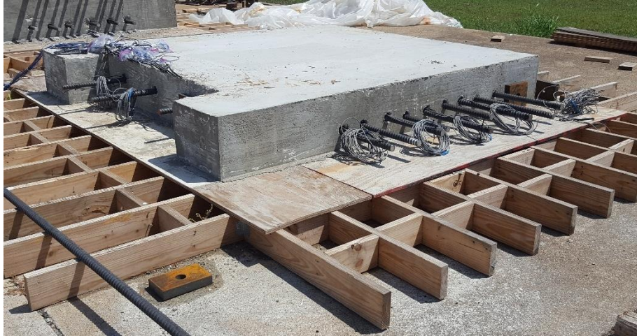
Figure 58 Specimen 1- Forms Stripped After Concrete Pour and Post-Tensioning Bars Installed
