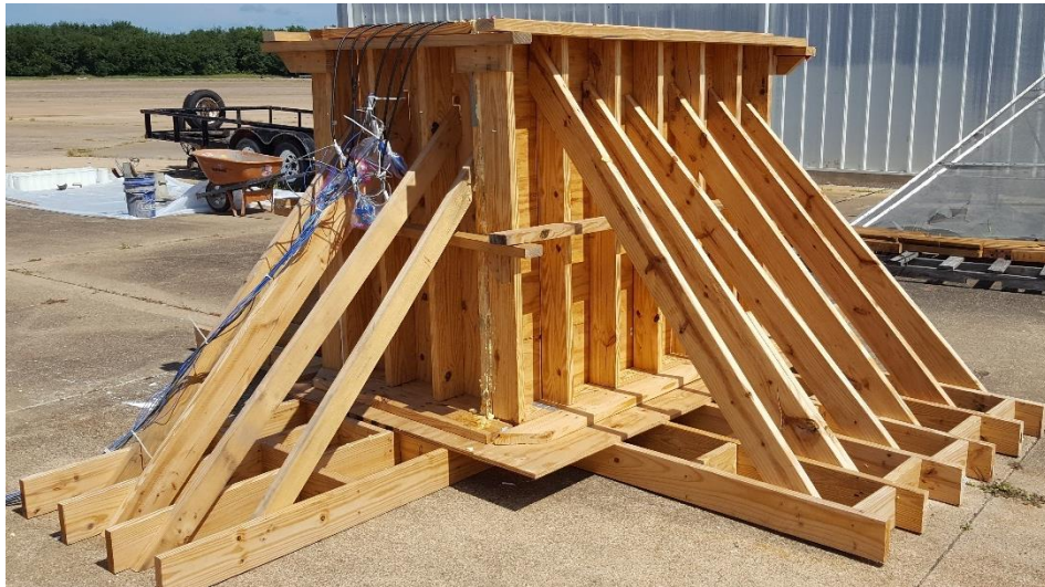
Figure 49 Specimen 3- Pre-Pour Set Up
