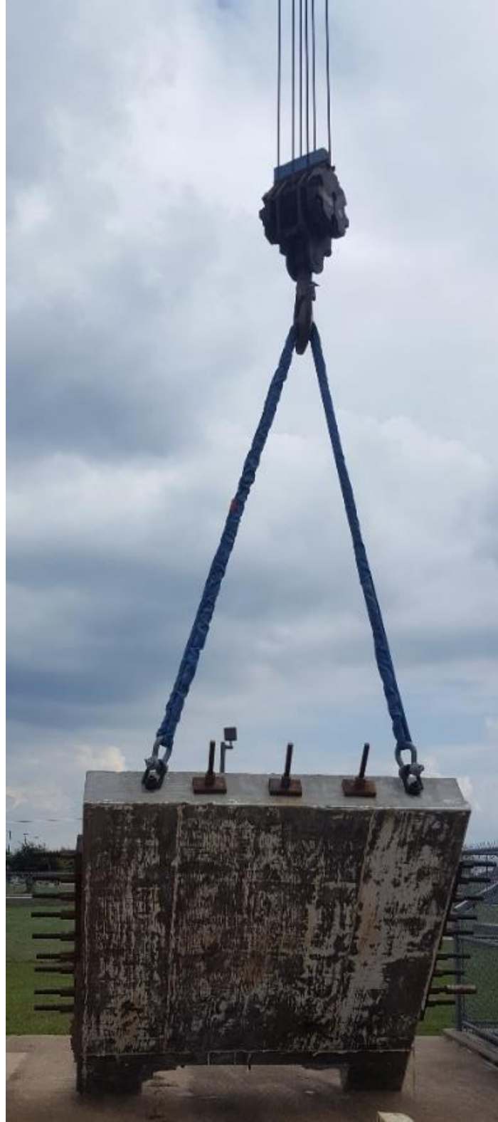
Figure 64 Specimen 1- Lifting Off Ground into Final Position
