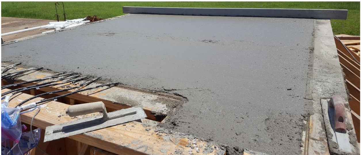
Figure 53 Specimen 2- After Concrete Pour
