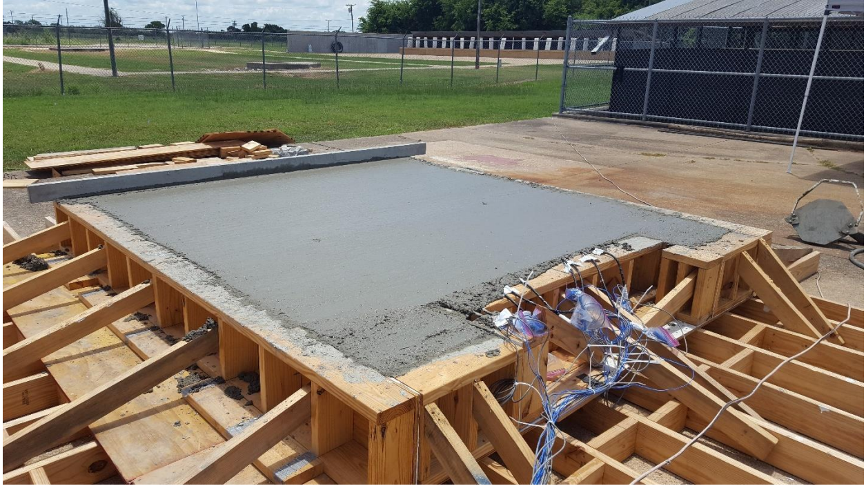
Figure 50 Specimen 1- After Concrete Pour
