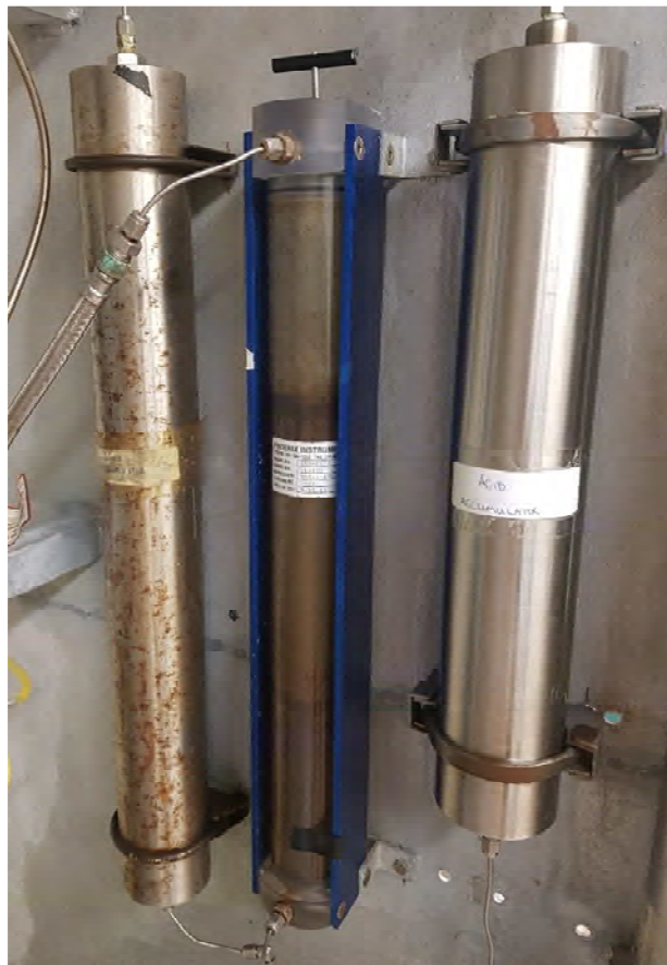
Figure 14. Acid (right) and water (left) accumulators with refill container (middle)
