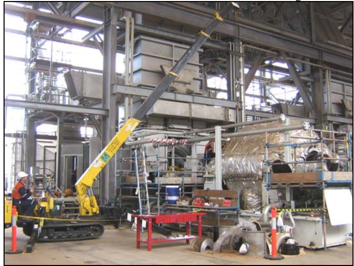
Figure 36. Propane Compressor Tertiary Seal Change out Activities.
