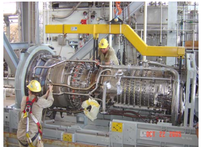
Figure 7. LM2500+ Gas Generator Being Installed.
