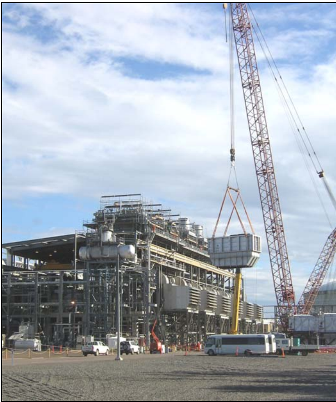
Figure 35. Change Out of OTSGs.
