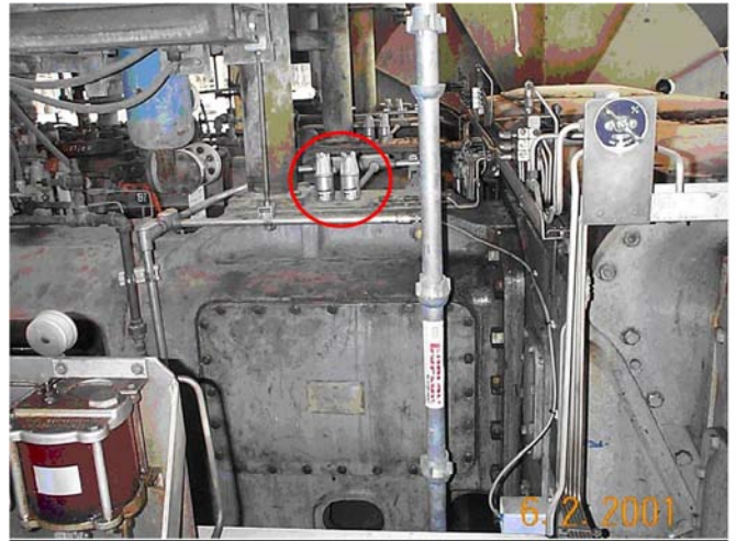
Figure 2: Crosshead Accelerometer installation. Courtesy of Bently Nevada.
