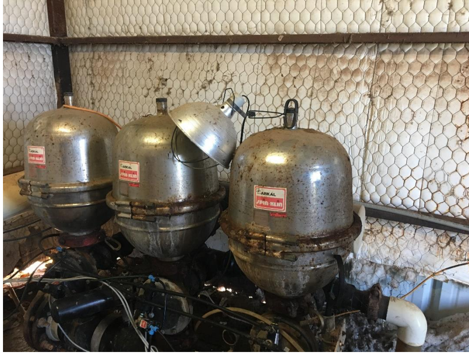
Figure 2: Treated wastewater disc filtration system: Amiad Arkal Spin Klin Filter. Filter has 120 mesh and 130 micron disc size.
