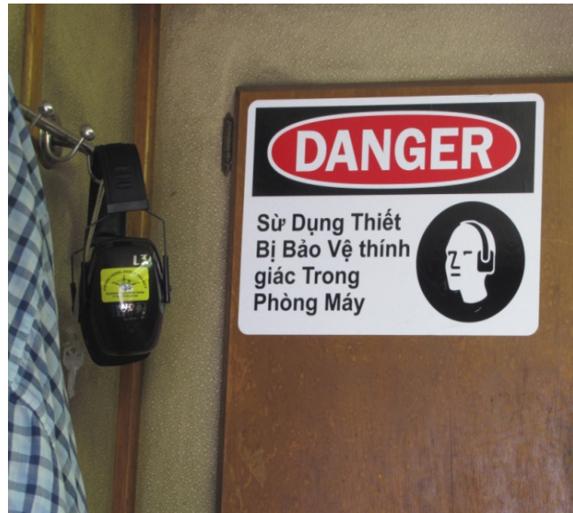
Figure 6.2. Noise warning sign in Vietnamese, at engine room. Note ear muffs.
