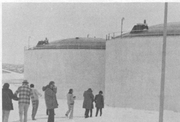
The 2-million-gallon anaerobic digesters at the Calorific plant near Guymon, Oklahoma daily convert 400 tons of manure dry matter into 1.6 million cubic feet of natural gas. Three similar plants are planned for the Texas Panhandle.
