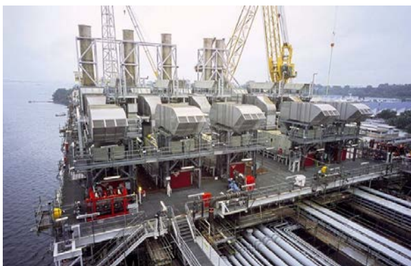
Figure 18. Gas Turbine Installation on an FPSO
