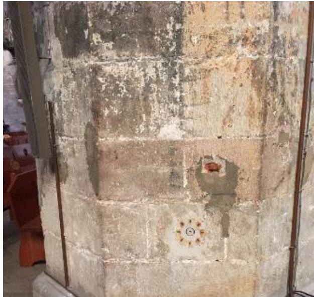
Figure 13: Color change on Pier 3 (note reds, yellows, and darkening)
