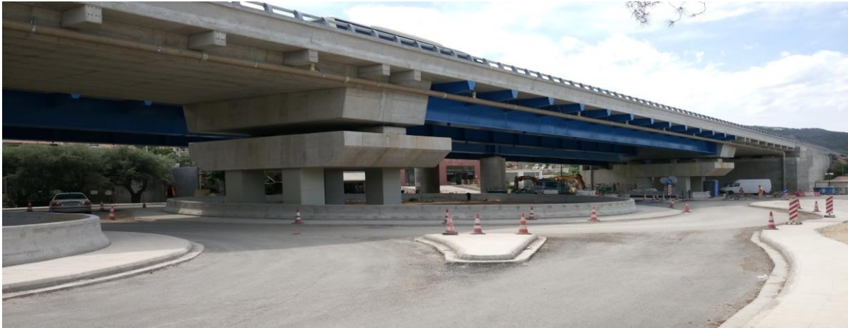
Figure 8.19 New Kamares Bridge after completion [© DENCO Structural Engineering P.C.]
