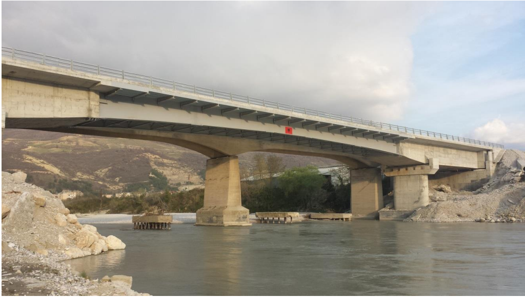
Figure 8.1 Memaliaj Bridge, Albania [© DOMI S.A.]
