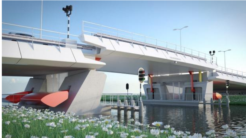
Figure 2.12 Nelson Mandela Bridge in Alkmaar (NL) FRP movable deck [Source: https://www.royalhaskoningdhv.com ]
