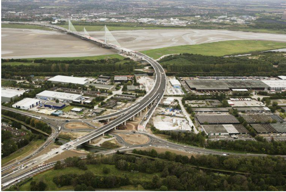
Figure 8.3 Astmoore and Bridgewater Bridge, United Kingdom [© DOMI S.A.]
