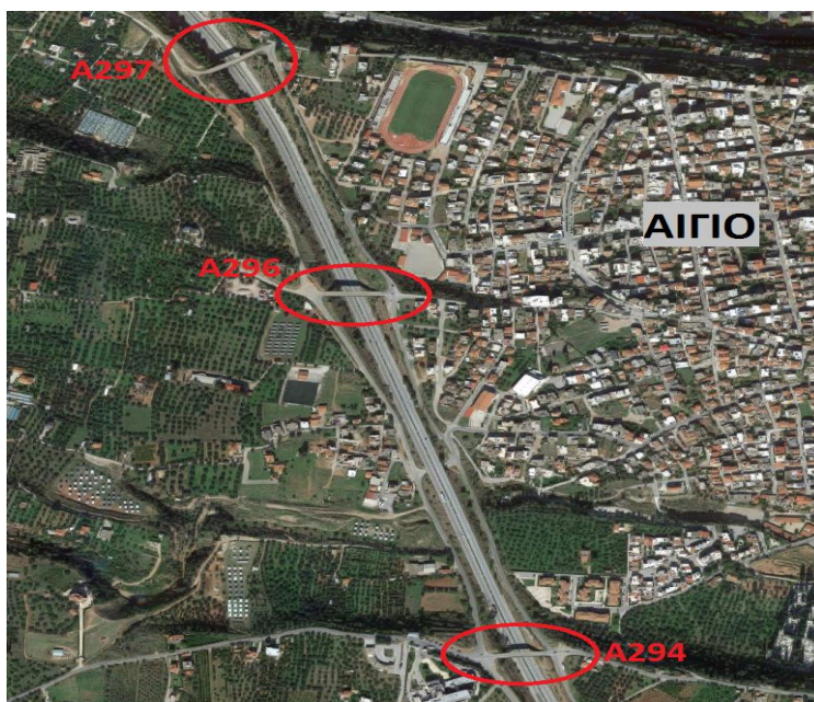
Figure 8.15 Location of Aigio Overpass Bridges, Greece [© DENCO Structural Engineering P.C.]
