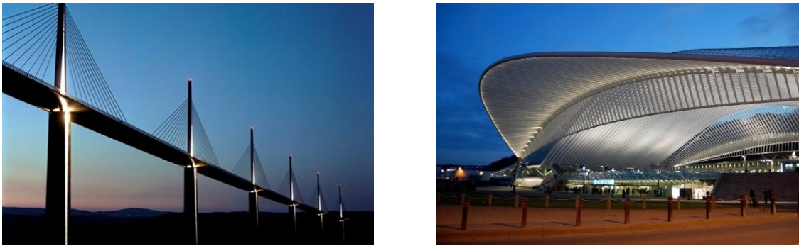
Figure 2.4 Examples of outstanding structures designed according to the Eurocodes [Source: (a) left: http://internal.schreder.com/en-au/projects/millau-viaduct © Schröder Group, (b) right: https://en.wikipedia.org/wiki/Li%C3%A8ge-Guillemins_railway_station ]
