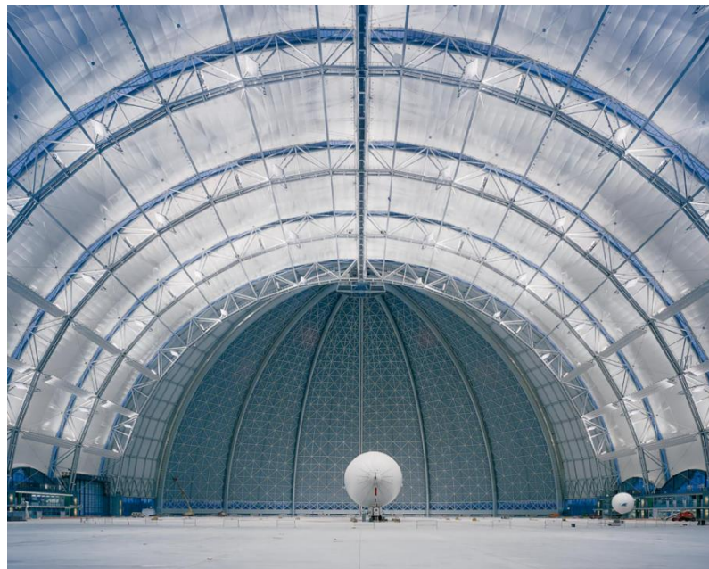
Figure 2.13 Cargolifter airship Hangar [Source: http://atlasofplaces.com/CargoLifter-SIAT-GmbH ]
