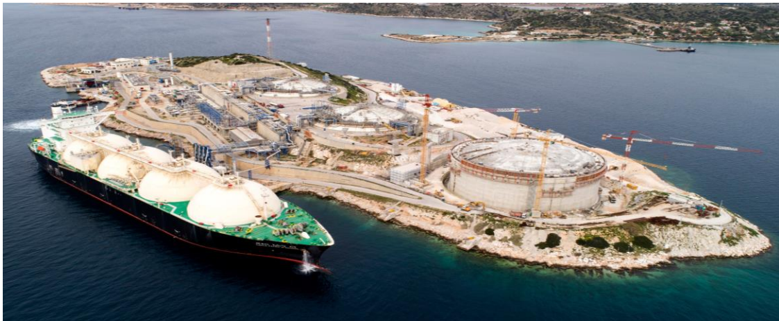
Figure 8.20 LNG plant in Revythousa island, Greece [© DENCO Structural Engineering P.C.]
