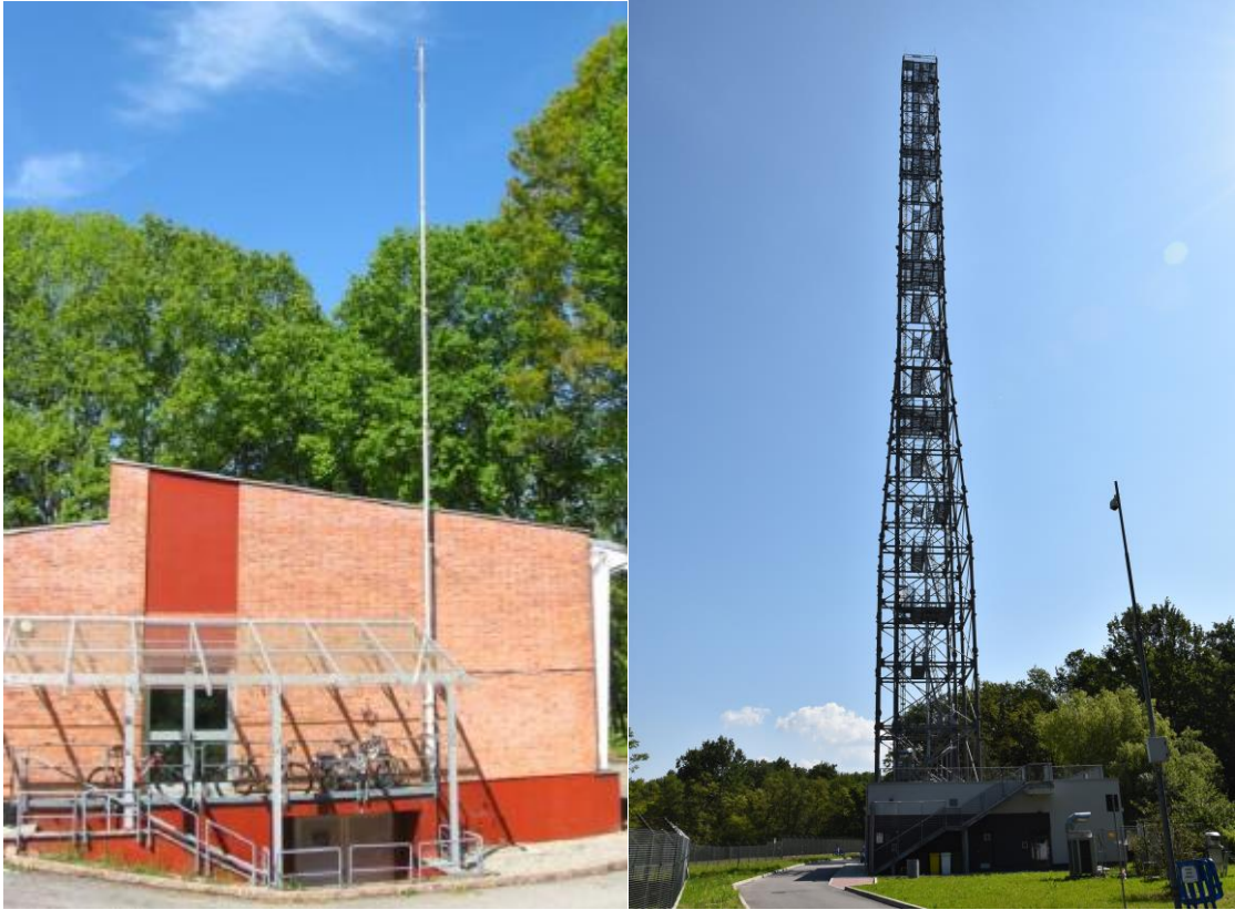
Fig. 2: The laboratories for atmospheric GHG measurements at Building 5 with 15m mast (left), and at the new JRC Atmospheric Observatory with the 100m-tall tower (Building 77r).
