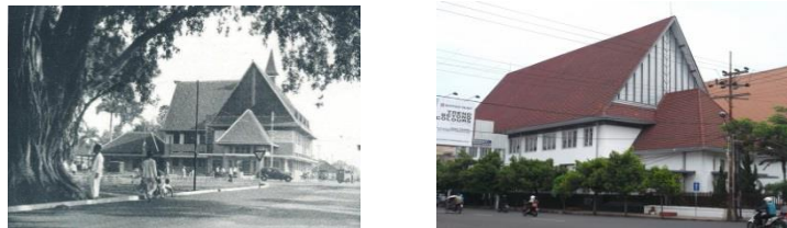
Fig. 2 (a) Office Of The Ministry of Treasury of Colonial Era, (b) Office Of The Ministry of Treasury of Colonial Era Today
