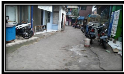
Fig.2. Building and Street Condition in Jalan Lada Dalam
