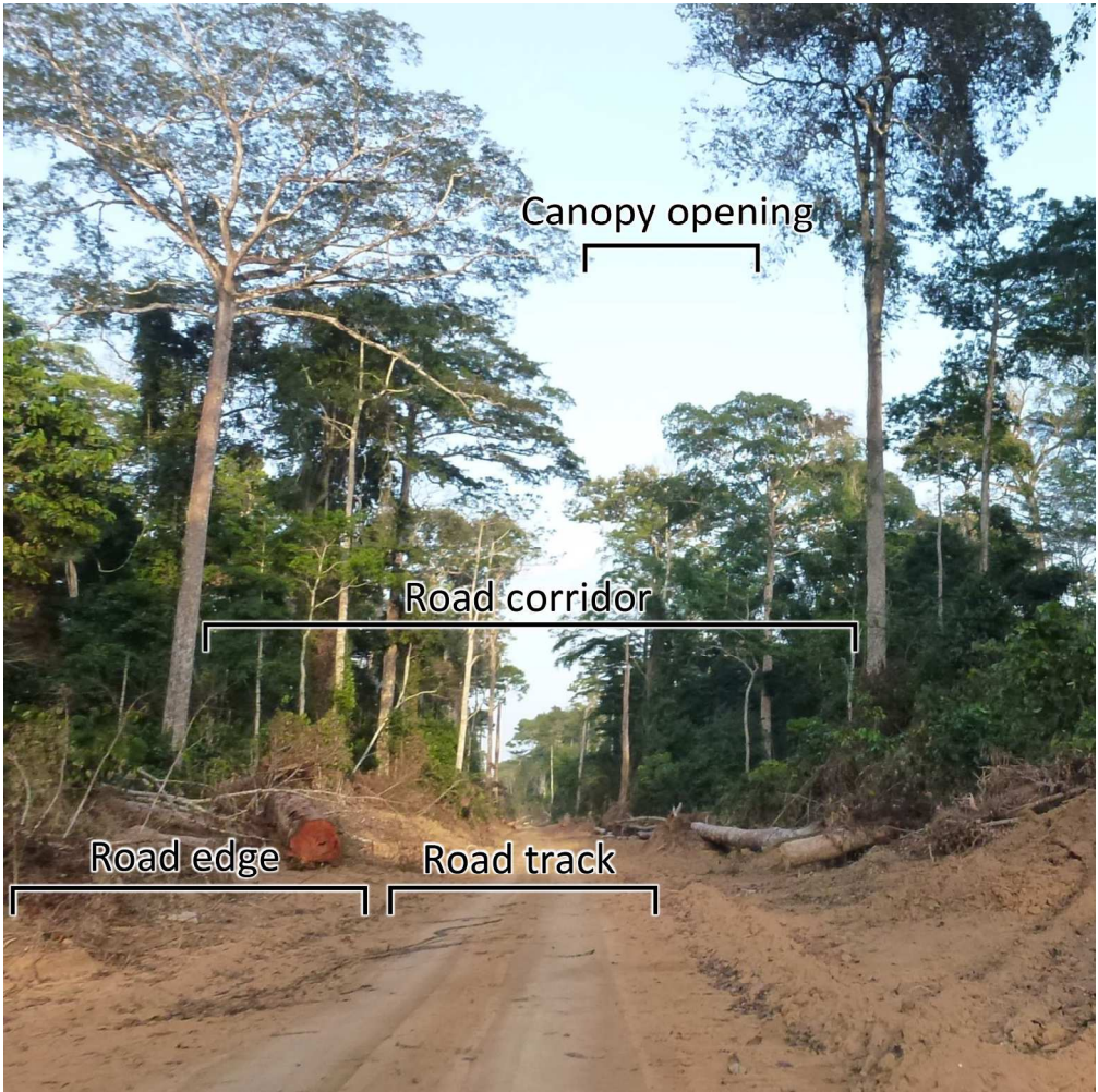
Example of a secondary logging road in Republic of Congo annotated with cross-section measures and their respective names used in the text.
