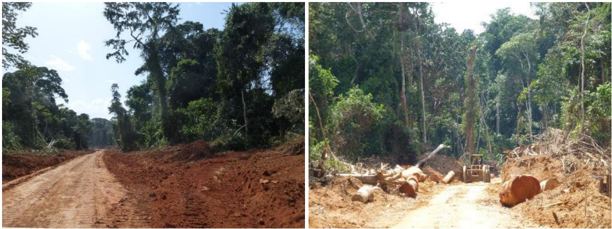
6 7 Figure 4. Newly constructed logging roads in south east Cameroon and northern Republic of 8 Congo. Left: Primary road making permanent access to the forest. Right: secondary (dead- 9 end) road built for temporary use to collect timber from log landings (here stored on the road 10 side).
