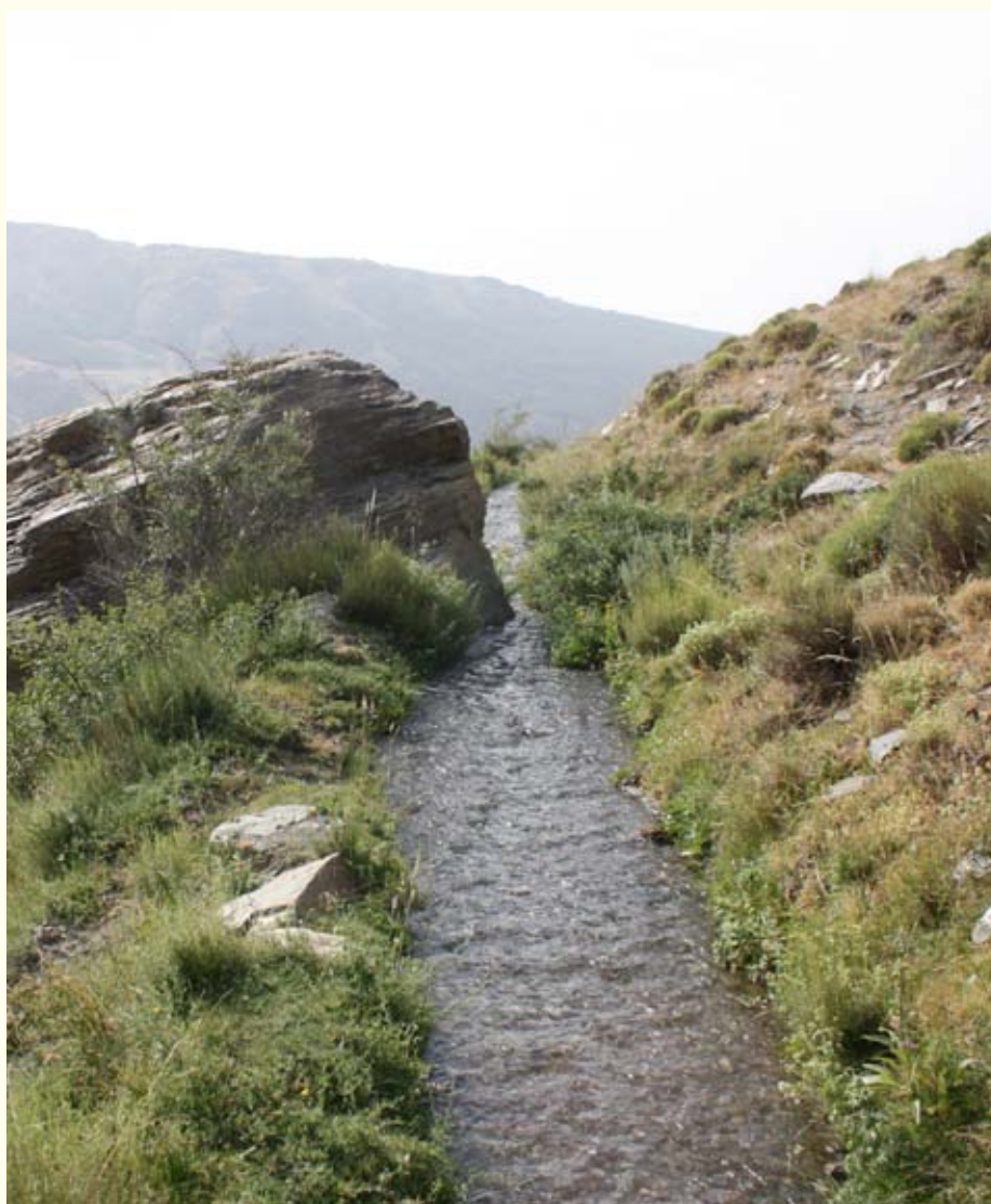
Traditional irrigation channel in Sierra Nevada
