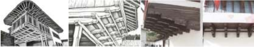
Figure 6. Wooden jetty drawings on the left (Doli, 2001) , the rest by the author
