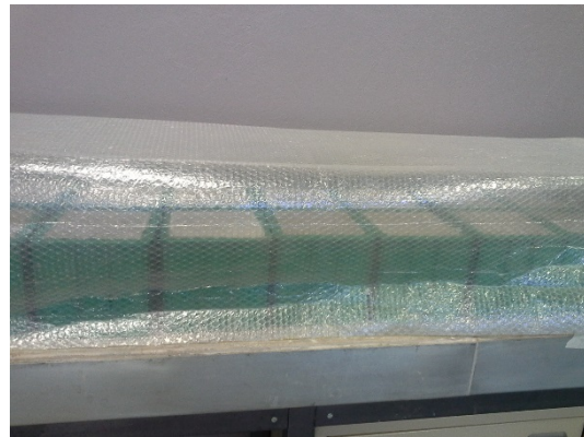
Concrete covered with polythene material
