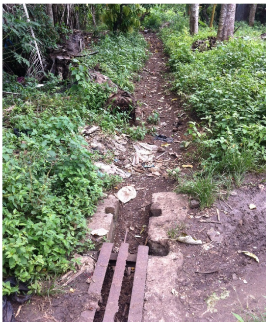
Picture 4. Old irrigation channel in Liberdade. Water flow is intermittent and depends on the water table in the nearby river.
