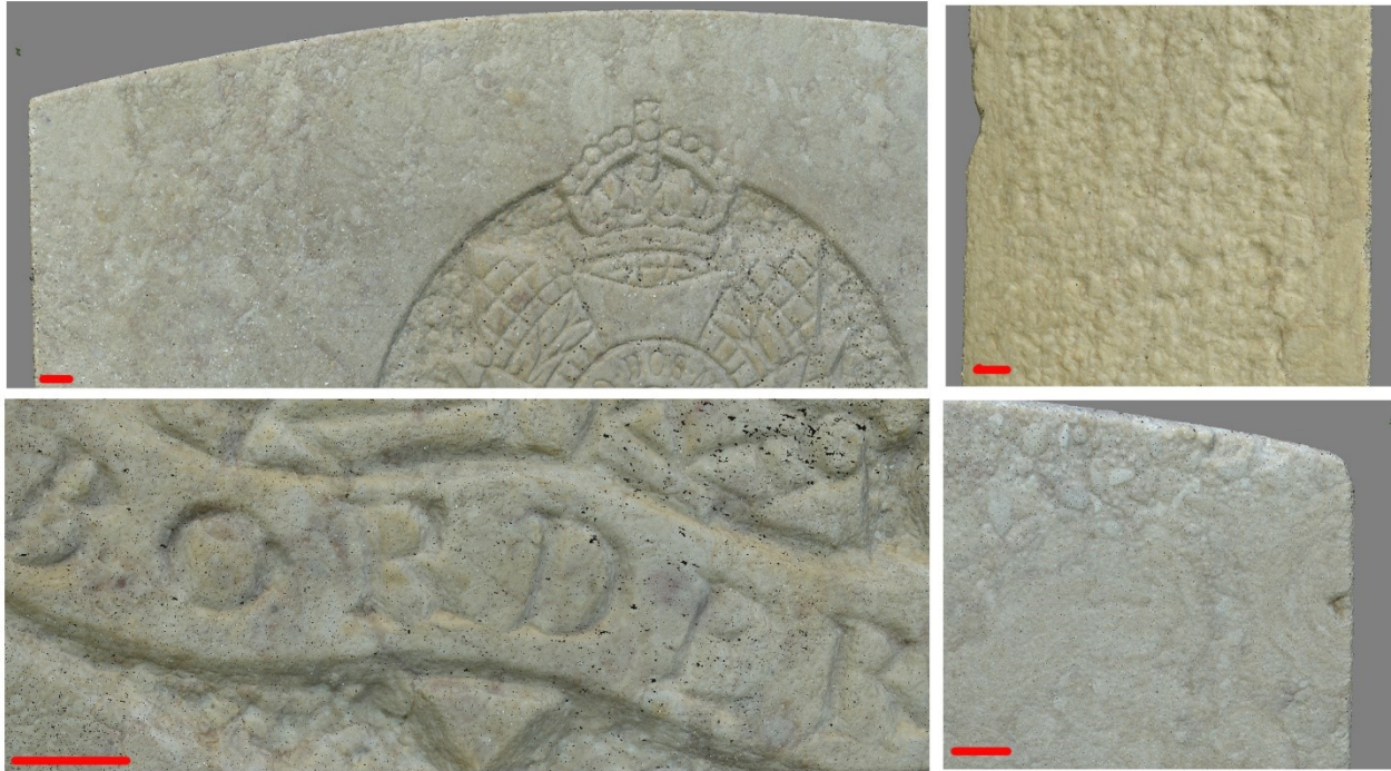
Figure 3. Details of the 3D model of the grave III.A.10 of the Bordighera British cemetery. This headstone is made of Chiampo stone and it is aged about 100 years. The red line stands for the unit of 1 cm.
