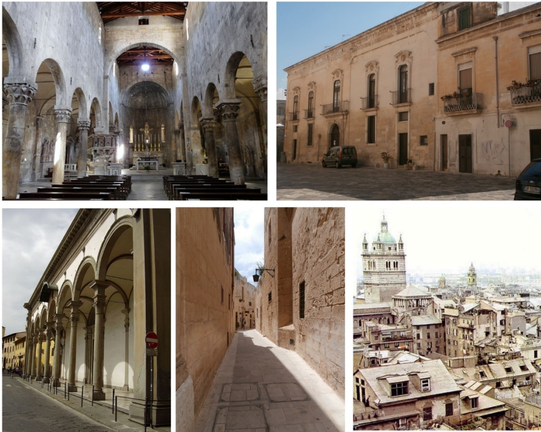
Figure 1. Views of old towns and historical monuments made with locally available stone building materials. From left to right: inside of the Carrara cathedral, totally covered with Carrara marble; street view of Lecce with buildings made of Lecce stone; view of a porch in Florence with columns and details made of Pietra Serena sandstone; town street in Malta with houses and urban paving made of local Globigerina limestone; view of the roofs of Genoa, covered with slate.
