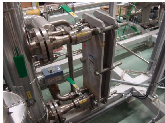
Figure 4.7 - Plate heat exchanger.
