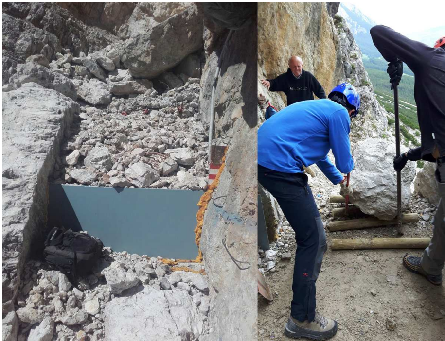
Figure 2.6: On the left, the situation found on the 27 th of August 2016 at the sharp-crested facility during an habitual reconnaissance; on the right, emptying of the basin like Egyptians.
