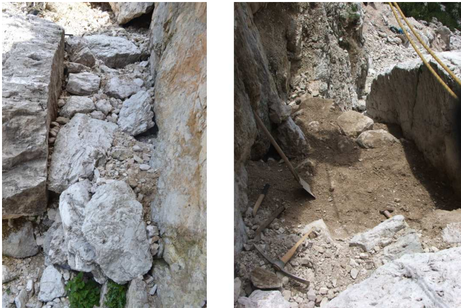
Figure A.1: Selection of the rocky channel for the setting up of sharp-crested weir (25 th of June 2011) and emptying.
