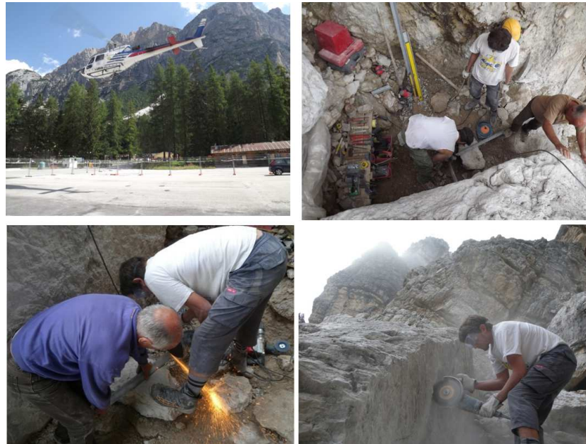
Figure A.2: Sharp-crested weir construction: initial operations (August 2011).
