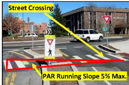
Figure 10: PAR Running Slope within Street Crossings
