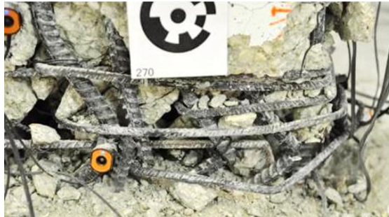
(a) Deformed confinement hoops
