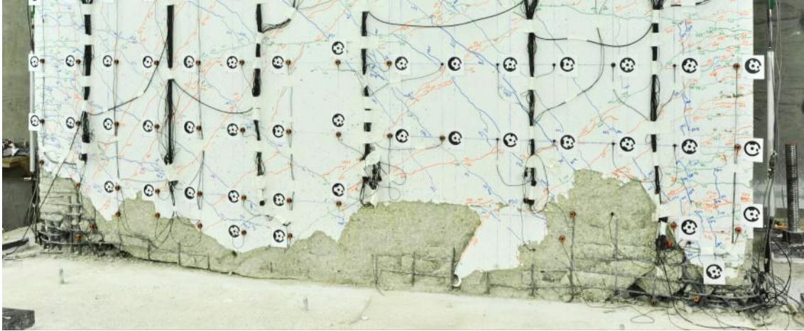
Figure 4.39: Photo of CW3 web crushing at the base of wall at the end of the test
