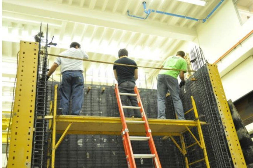
Figure 3.7: Nearing completion of CW3 rebar cage
