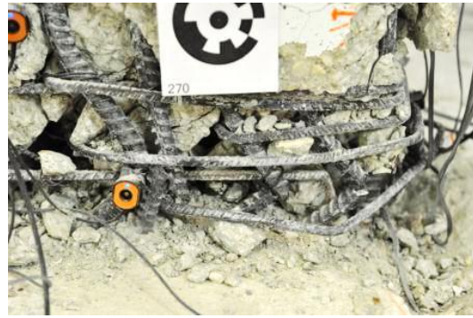
(b) Southeast corner
