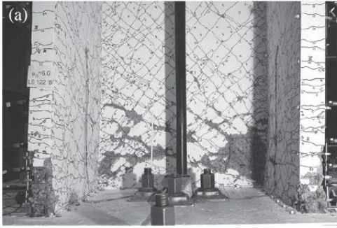
(a) Photo of interior of U-shaped wall web
