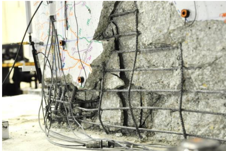
Figure 4.41: East flange damage attributed to out-of-plane shear demand in CW3
