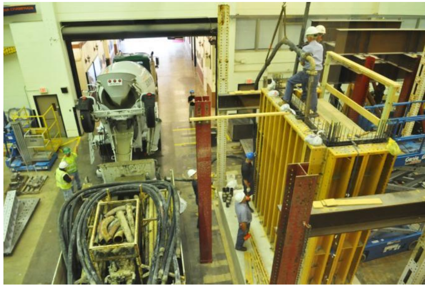
Figure 3.8: Casting of CW3 specimen
