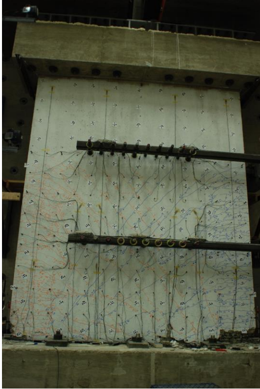
(a) Photo of cracking and damage
