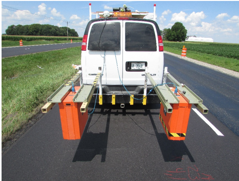
Figure 7-5 GPR static data collection on US Route 45 after leveling binder was placed
