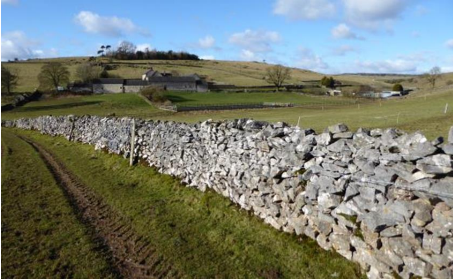
Late 18th century enclosure wall, looking east towards the 18th-19th century farmstead at Roystone Grange, and the Romano-British enclosures on the rising land behind it.
