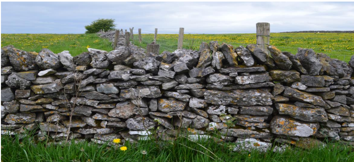
Straight joint indicating the phasing of dry stone walls in an area of former wastes and commons enclosed in the early-mid 19th century enclosure
