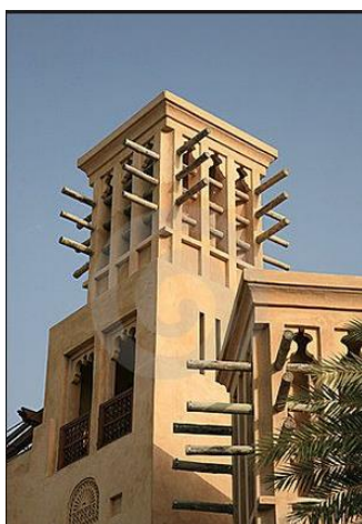
Figure 3.12: Building materials and roofing system
