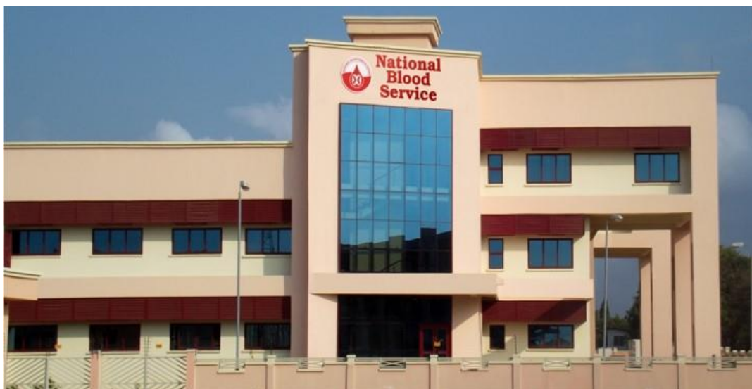
Figure 1-1: The front view of the NBSG Headquarters and Southern Area Blood Centre
