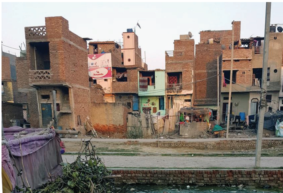
Figure 1. A typical street and the range of dwellings found in the resettlement colony, Savda Chevra.
