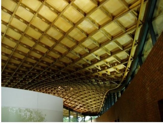
Figure 13: The Savill Garden gridshell completed in 2005 was restrained by a double layer of plywood working in shear. [Photograph © Gabriel Tang]
