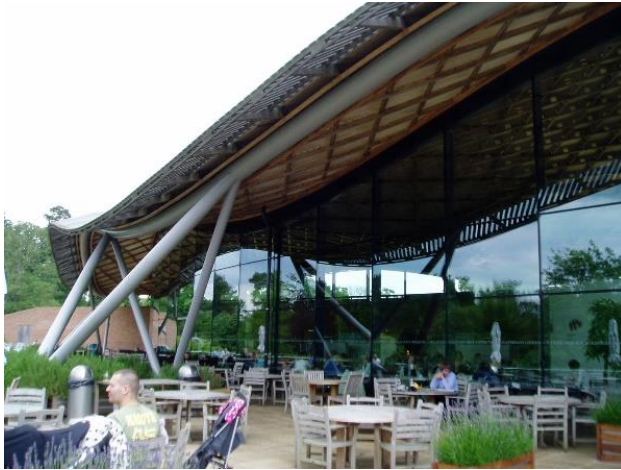
Fig 15: The Savill Garden gridshell, completed in 2005, is raised above ground by 8m long steel columns and the shallow gridshell structure is restrained by a 400mm diameter tubular ring beam. [Photograph © Gabriel Tang]
