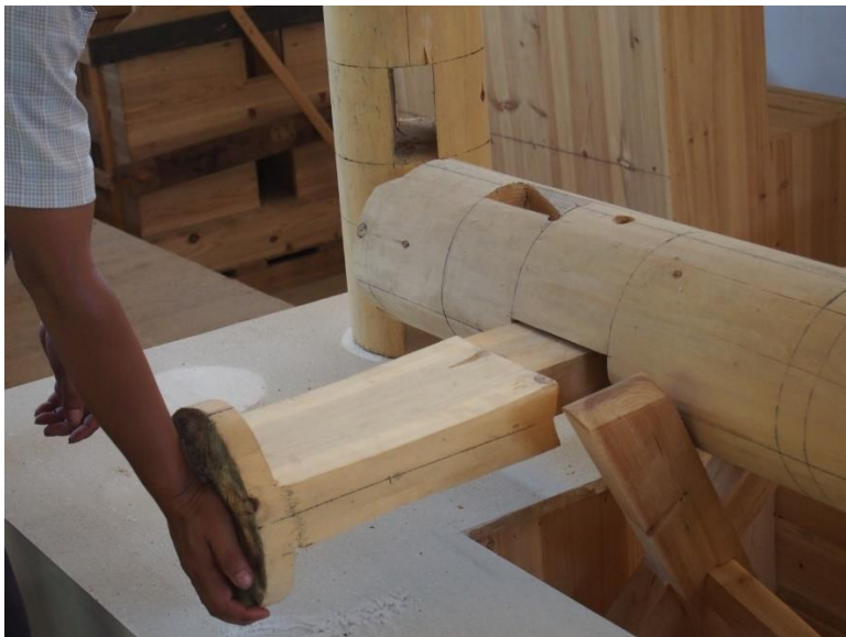
Figure 5: Traditional tenon and mortise joints, Maogong, China [Photograph © Gabriel Tang]
