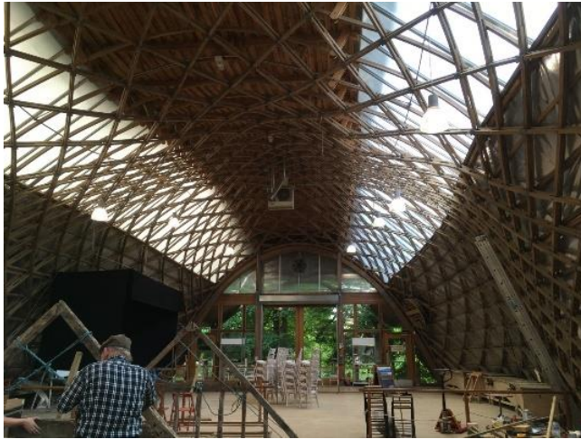
Fig 10: The Weald and Downland Jerwood Gridshell, Singleton, Chichester, UK designed by Studio Cullinan and constructed by Green Oak Carpentry Company 2003 [Photograph © Gabriel Tang]
