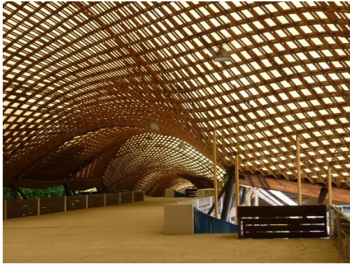
Figure 11: Mannheim Multihalle was created by pushing up gridmats from the ground [Photograph © Gabriel Tang]
