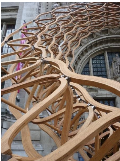
Figure 8: The Timber Wave Sculpture designed by Amanda Levete Architects and constructed by Cowley Timberworks, Victoria and Albert Museum, London, UK, 2011 demonstrates the expression of metal fastenings and fitch plate connections. [Photograph: © Gabriel Tang]
