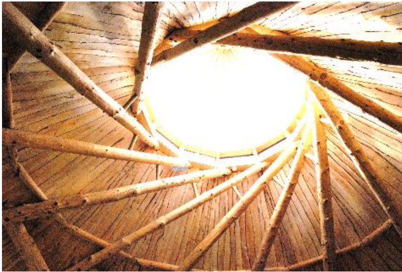
Figure 3: Reciprocal frame timber roof at Hill Holt Wood, near Newark, UK, assembled from CNC machined tree trunks [Photograph © John Chilton]
