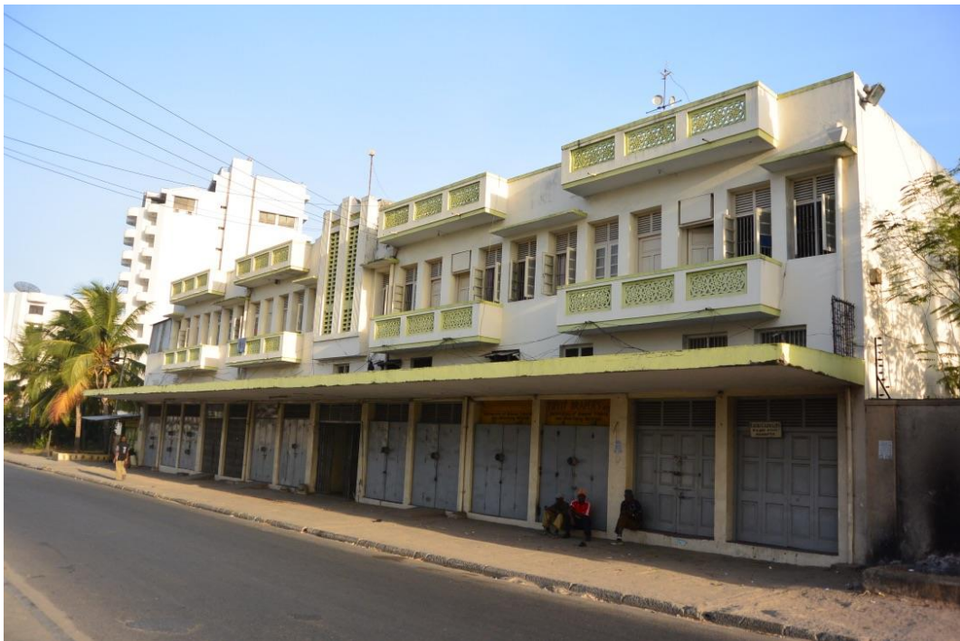
Figure 20: White and green Art Deco apartments with commercial premises below, Mwembe Tayari Road.
