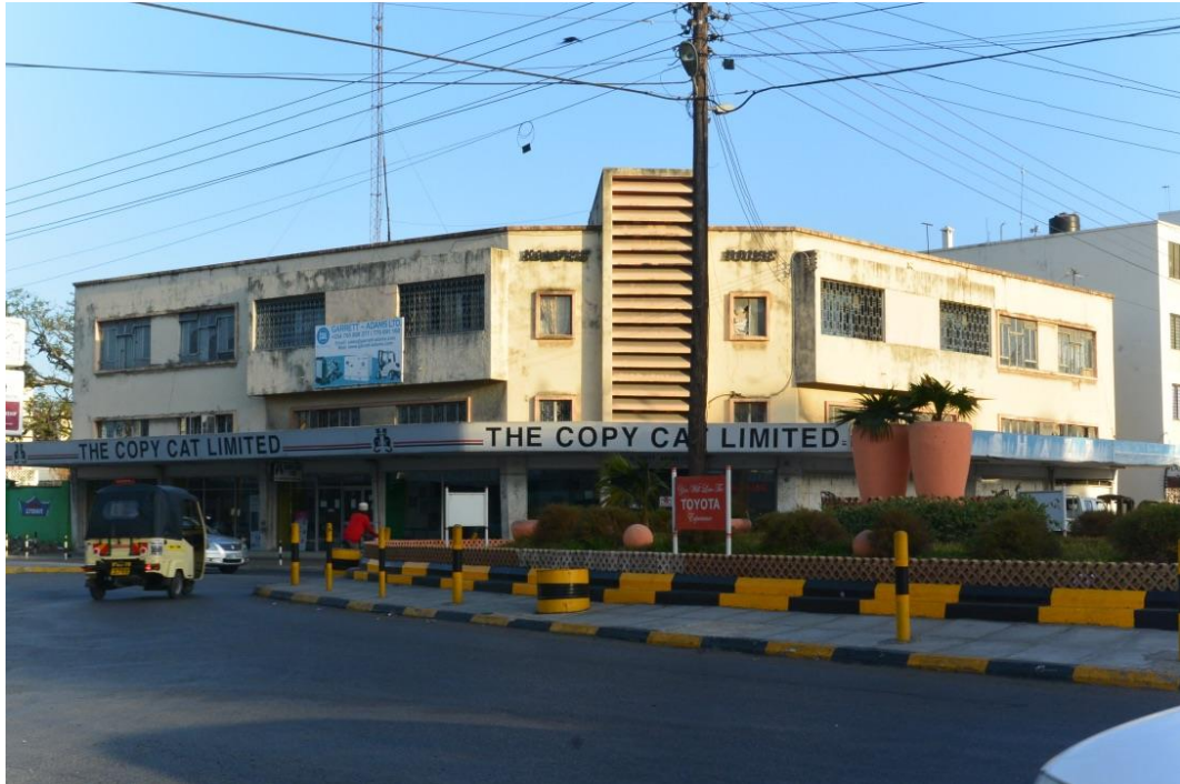
Figure 19: Kampee House, above the Copy Cat Limited, Moi Avenue. An oversized ventilation grill forms its central pillar.
