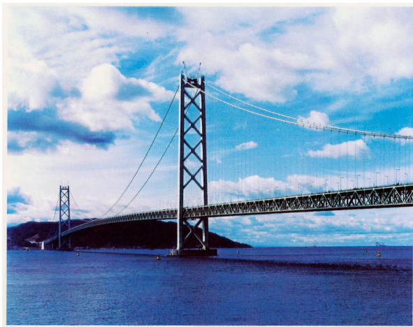
Figure 1. The Akashi-Kaikyo Bridge in Japan, the longest single-span suspension bridge, which relies on huge cables made from pearlitic steel. Photograph courtesy of Professor Nobutaka Yurioka.
