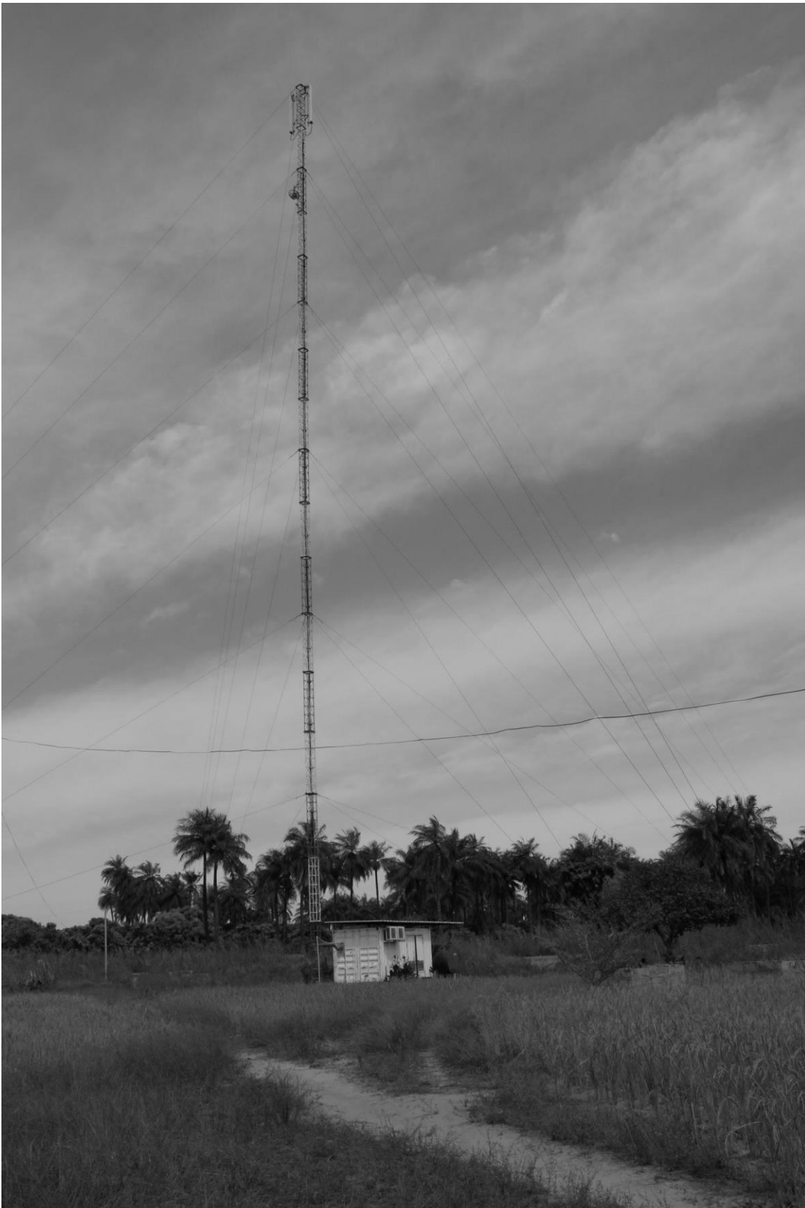
Fig 1. Off-grid mobile phone receptor mast powered by a diesel generator.
