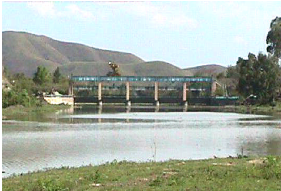
Figure 2.37. Ithai Barrage looking downstream
