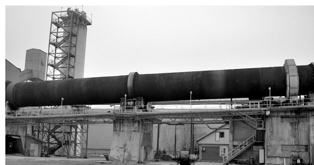
Figure 1 Rotary kiln in the cement plant in Kakanj
