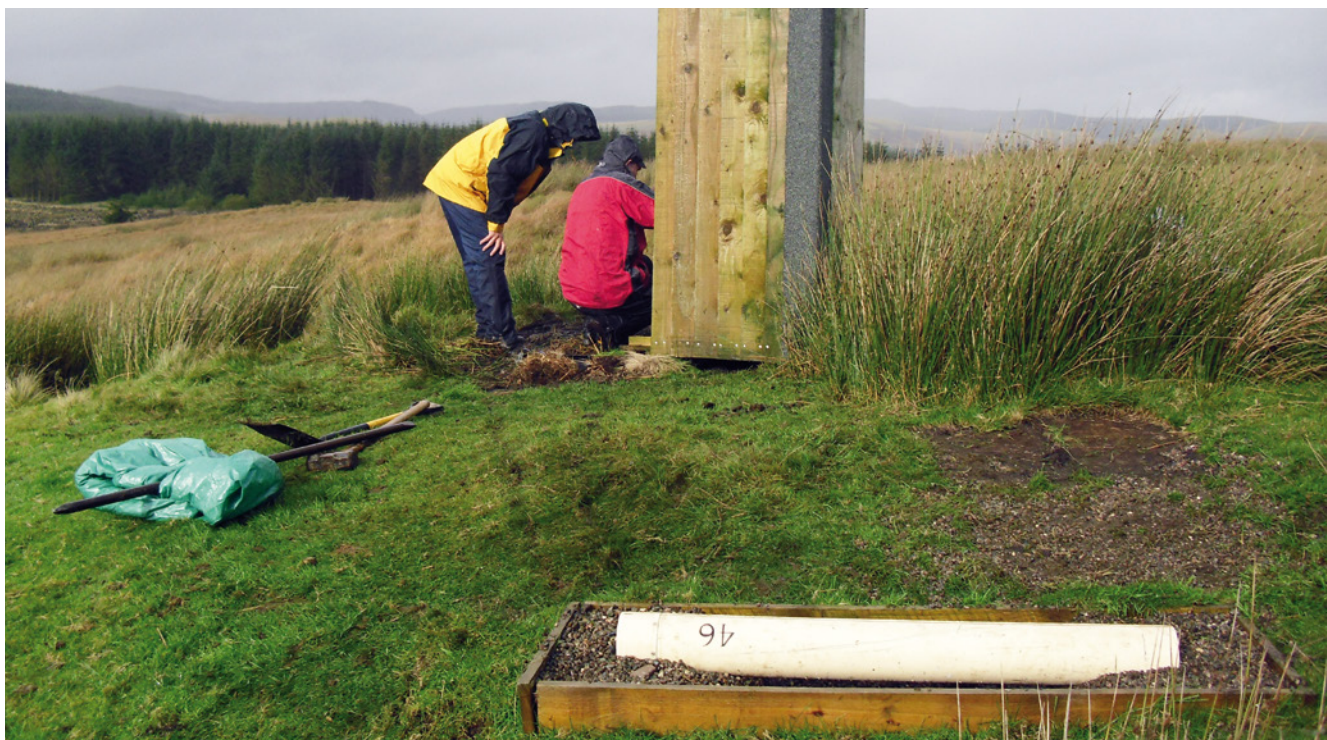
Members of the Geomagnetism team link an induction coil to a nearby break-out box and digitiser at Eskdalemuir. The induction coil is placed on a levelled bed of gravel.
