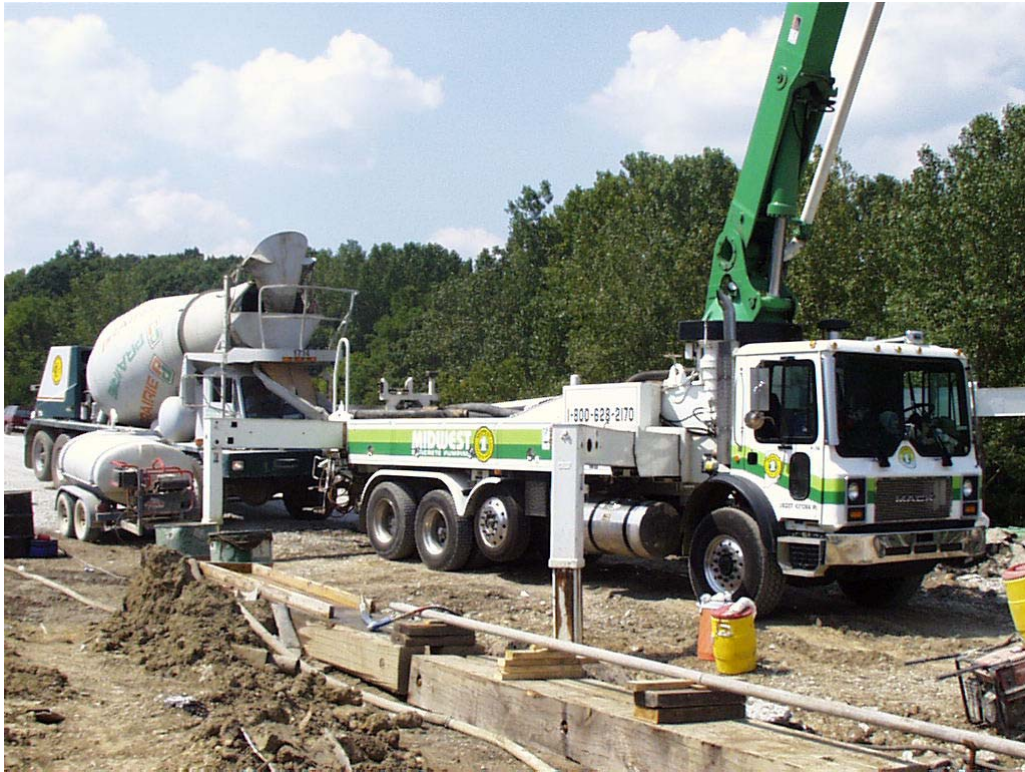
Figure 137. Concrete pumping operation
