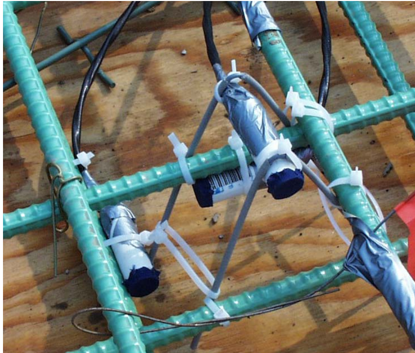
Figure 140. Internal RH sensors mounted for casting in concrete bridge deck
