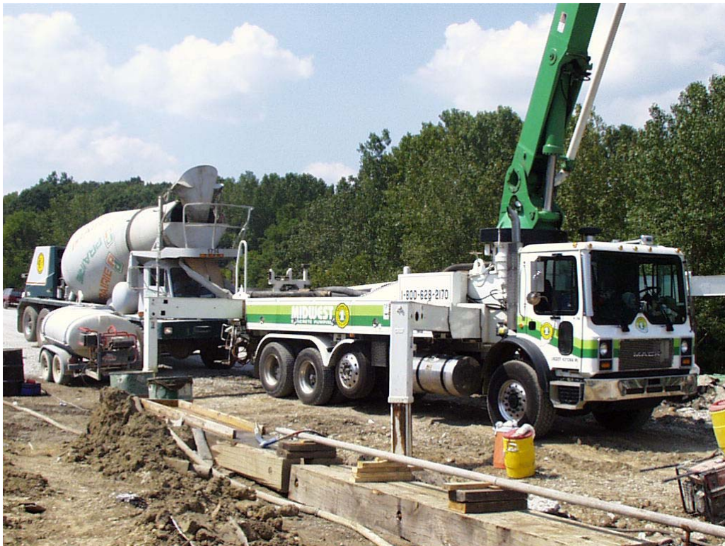
Figure 239. Concrete pumping operation, Big Creek
