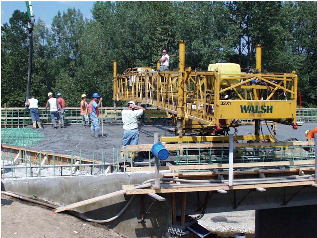
Figure 138. Placing and finishing concrete
