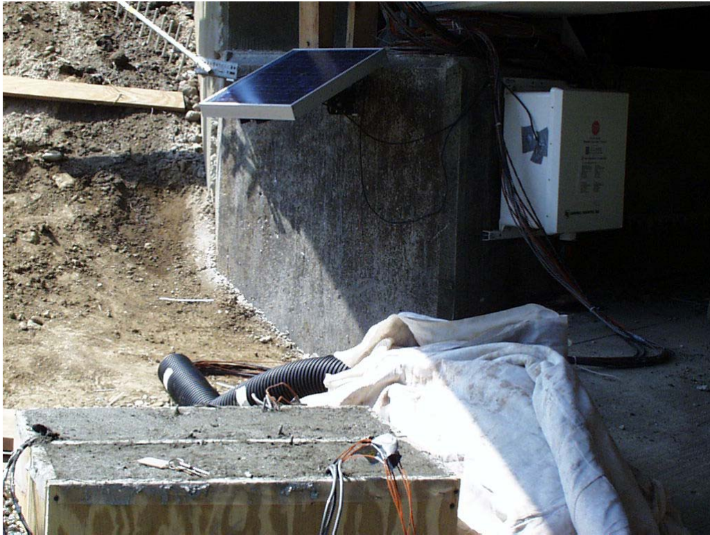
Figure 238. Data collection system and free shrinkage beams, Big Creek
