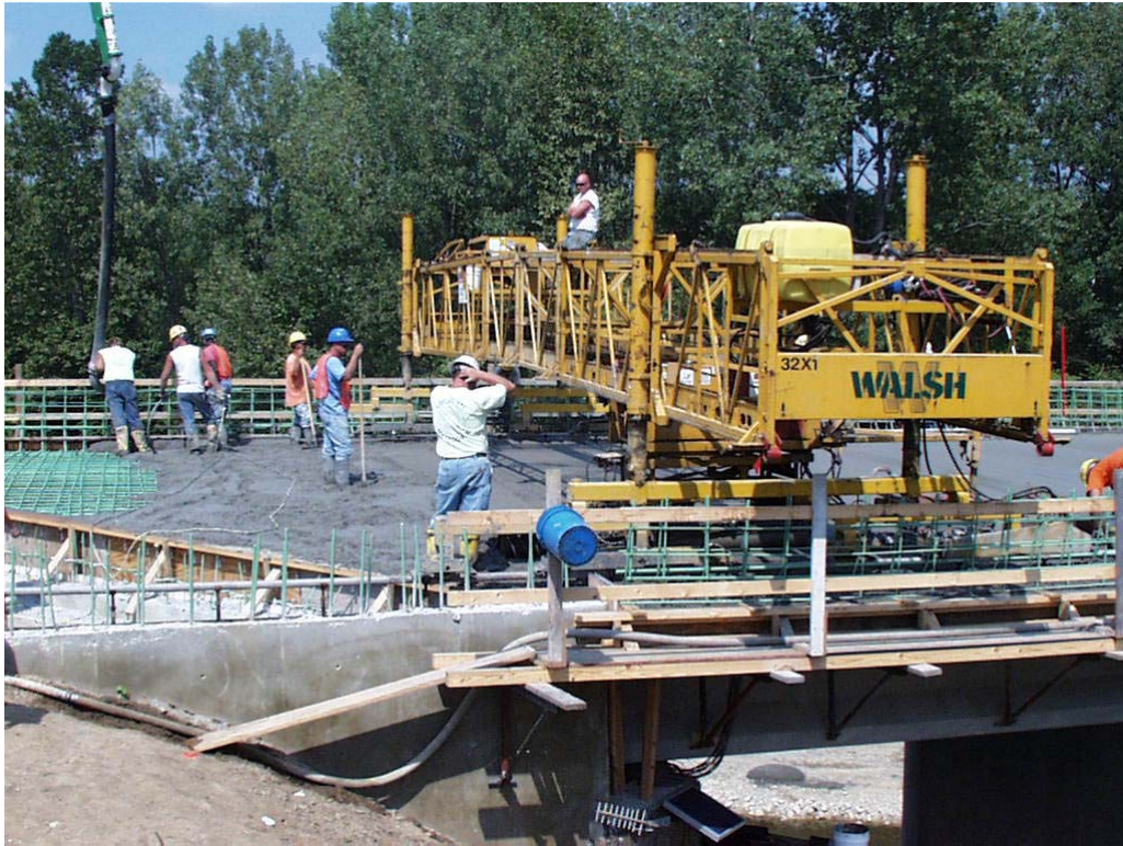
Figure 240. Placing and finishing concrete, Big Creek
