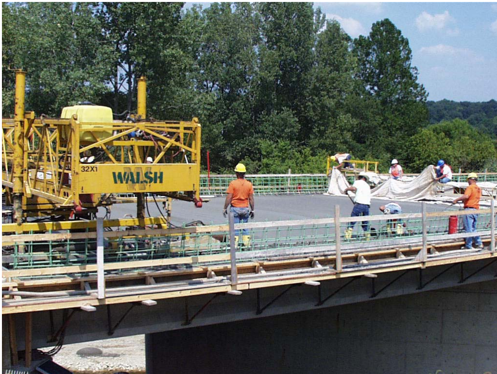
Figure 241. Applying wet cotton mats for curing, Big Creek
