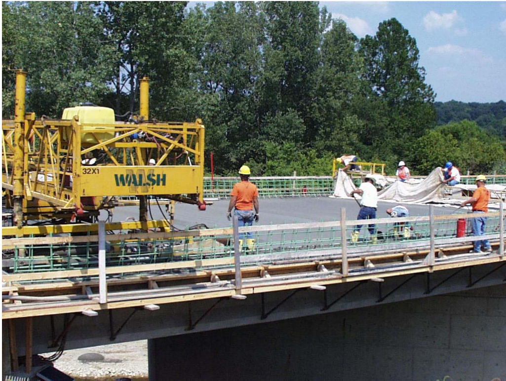
Figure 139. Applying wet cotton mats for curing
