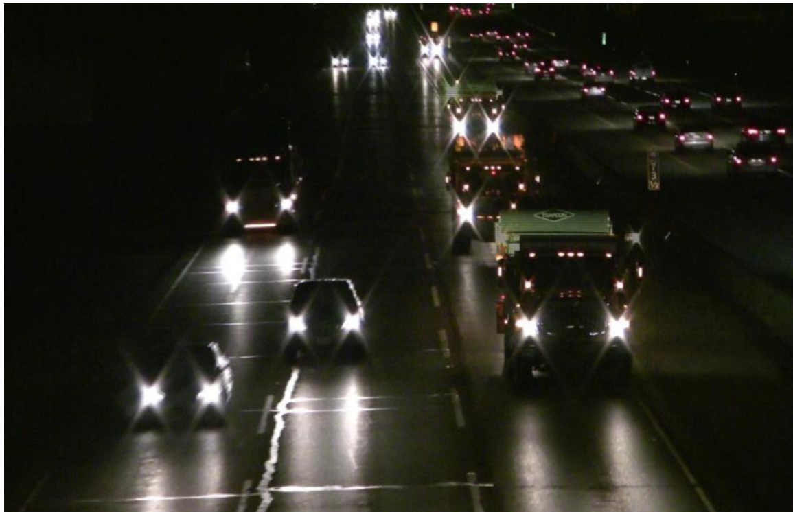
Figure 4.6 Lateral lane positions for the mobile lane closure near the Des Plaines Oasis. Vehicles driving in the center of the lane with all lanes open (top) and a vehicle in the center lane shifting away from the traffic control operation (bottom).
