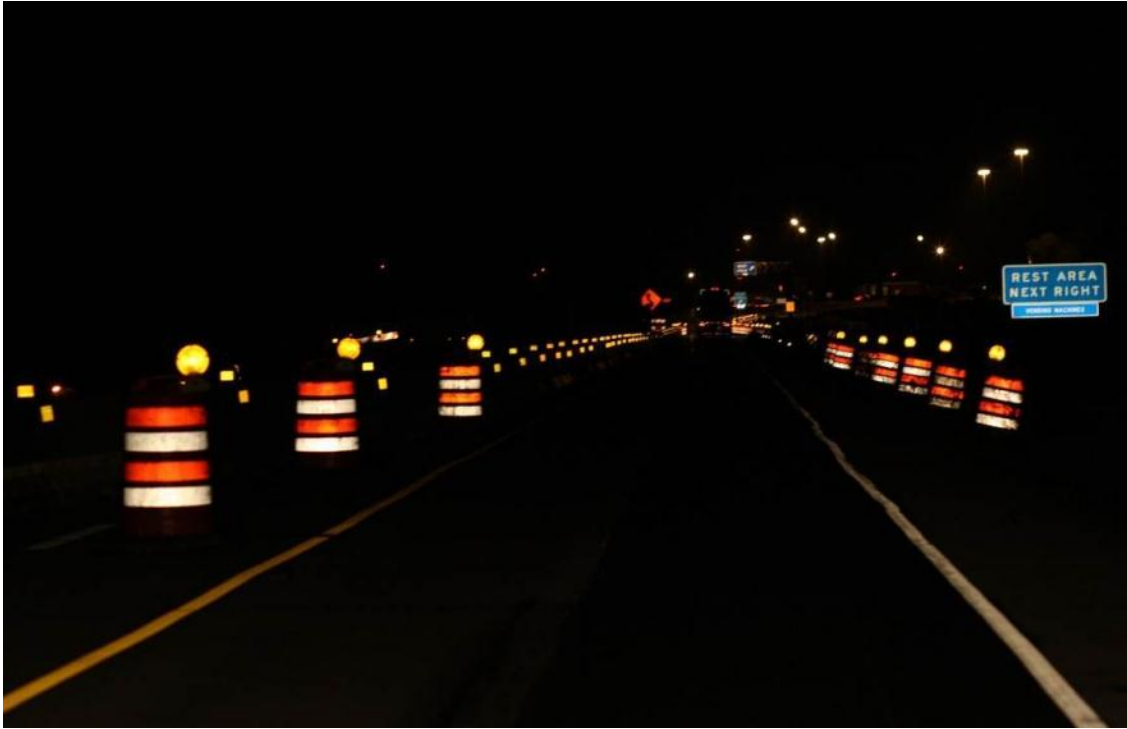
Figure 6.10 A left-lane closure on I-57 near Buckley because of bridge construction. Traffic has merged to the right lane and partially shifted on to the shoulder. No workers are present.
