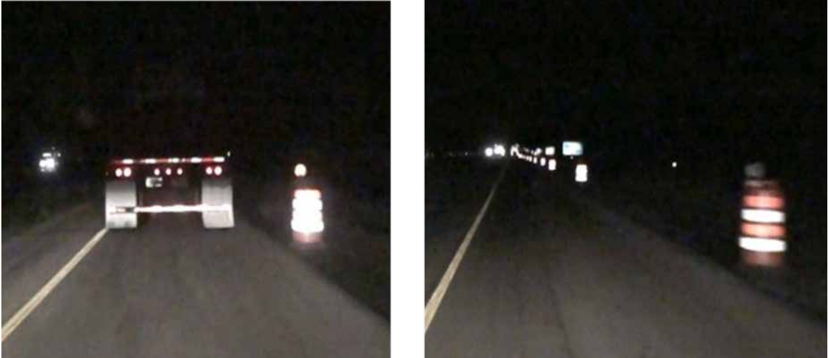
Figure 4.10 Driver's perspective of the lane closure for the lights-on and lights-off conditions downstream of the paving operation, Salem site.
