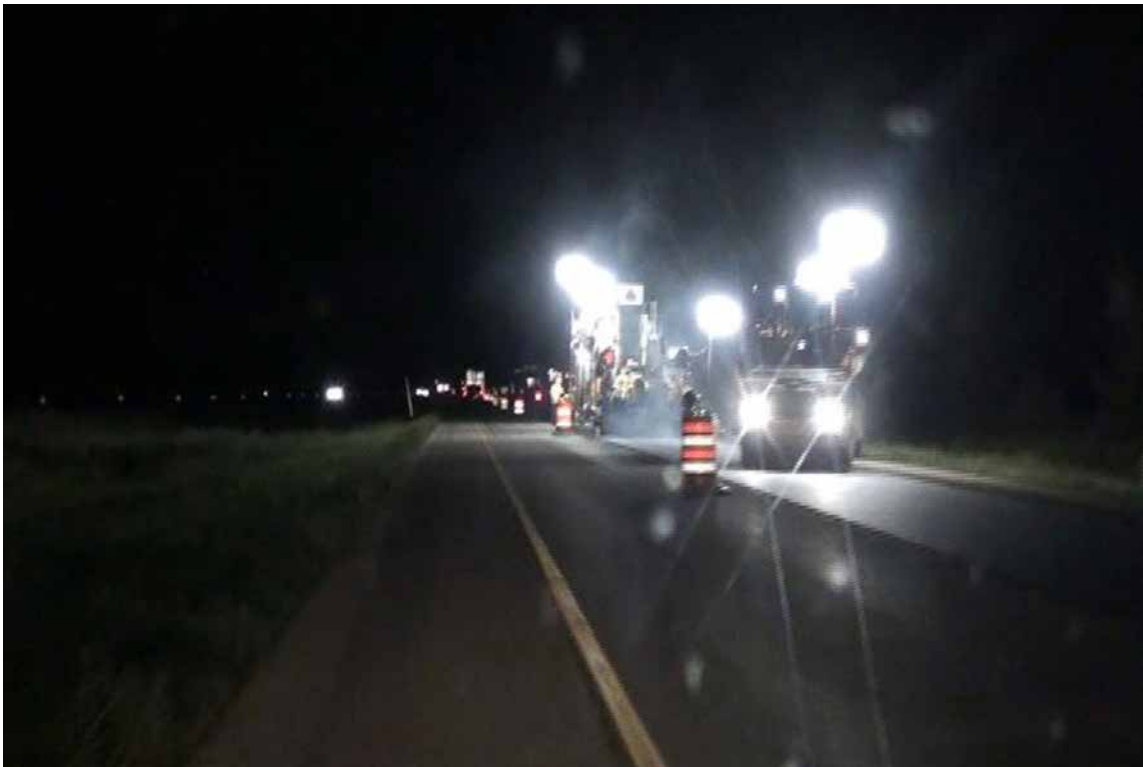
Figure 4.9 Overview of the Salem test site showing the nighttime paving operation.
