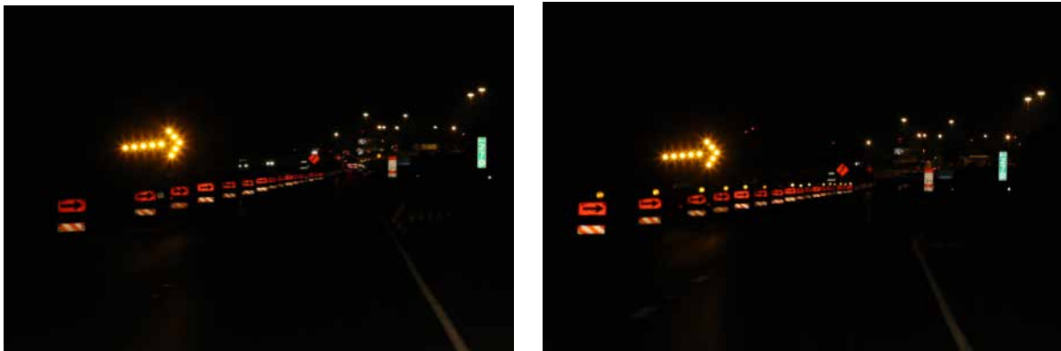
Figure 4.2 Taper with lights off and lights on directional barricades at the Buckley site.
