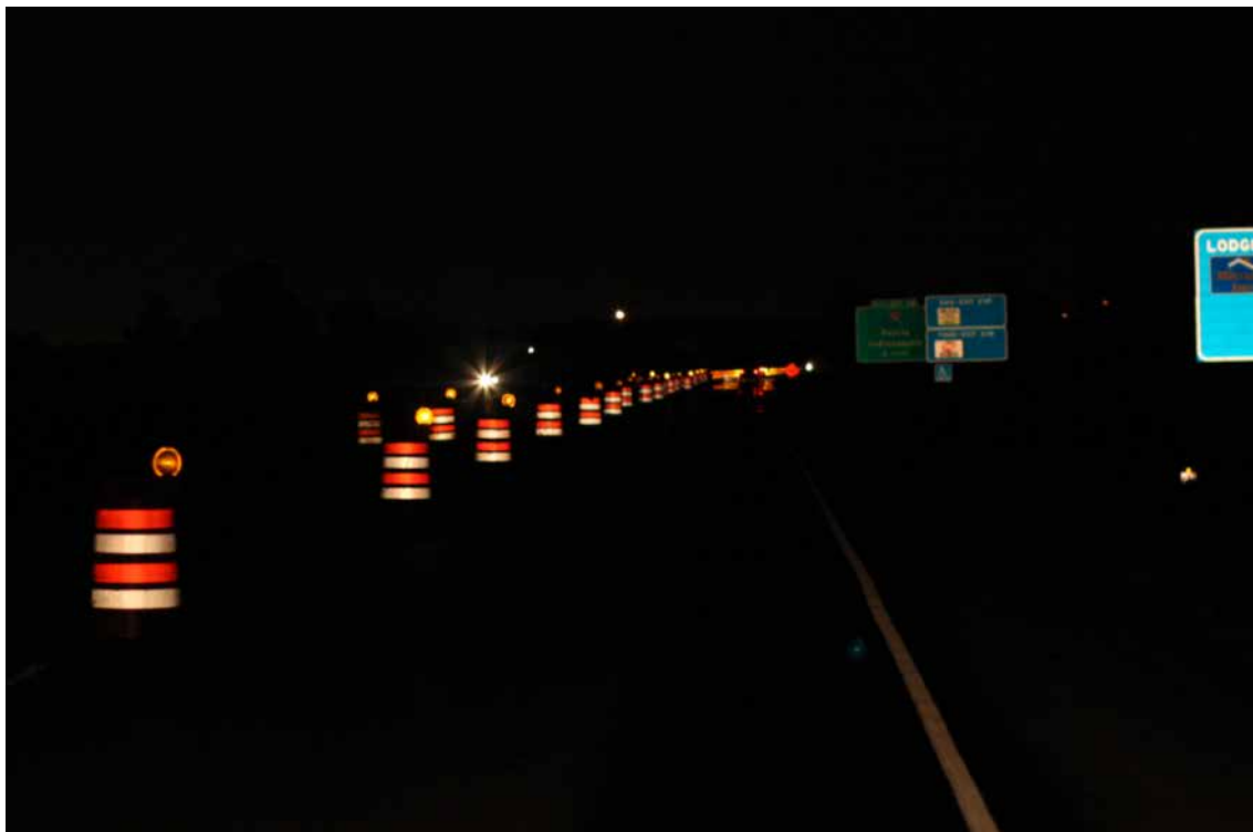
Figure 6.11 A left-lane closure on I-57 near Champaign. Traffic has been merged to the right lane, and no workers are present.
