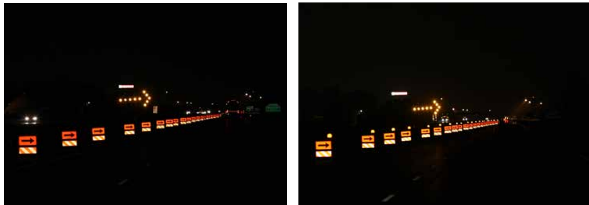
Figure 4.5 Taper with lights off and lights on direction indicator barricades at the Champaign site.
