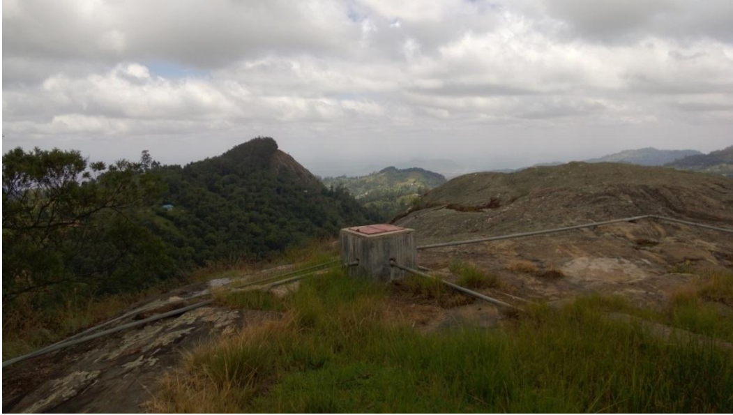
Figure 25 In many cases the maintenance falls on the community members themselves, who might not have the technical knowledge or tools to repair the water infrastructure. These pipes on the top of Kiangungu hill were leaking and a group of drunken men came to fix it since their village had been without water for 3 weeks. (Kivivuori 2013)
