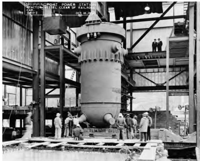
Figure 3.4: The RPV of the Shippingport Atomic Power Station, PA, USA, during transportation in 1956 [12].
