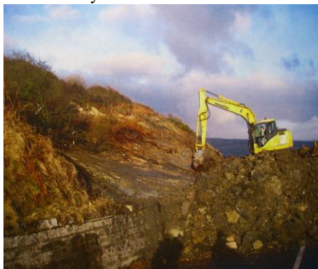
Figure 1. Landslide debris on A2 Coast Road, 25 th January 2010
