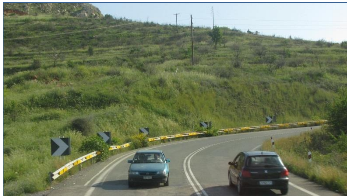
Figure 3. Panels of retroreflective sheeting to delineate curves
