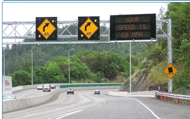
Southbound signs before and after
