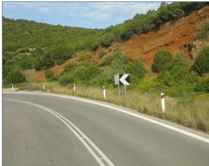
Figure 20. Post delineators on a curve
