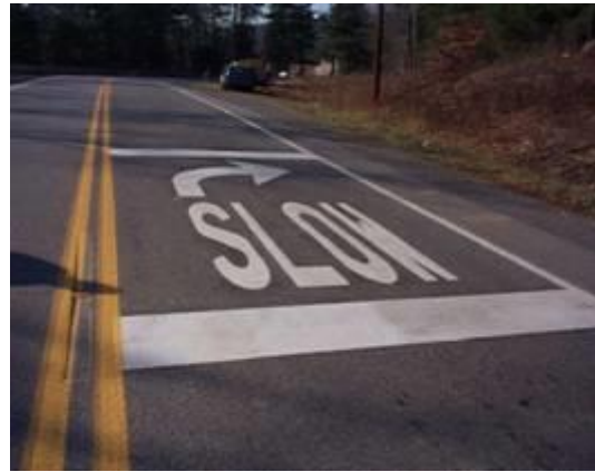
Figure 32. On-pavement treatment applied in Iowa
