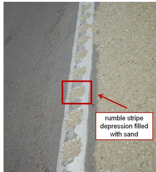
Figure 29. Rumble stripe depression filled with material (Hallmark et al. 2011)
