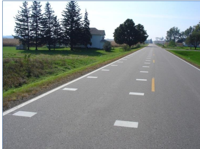
Figure 12. Transverse pavement markings as a rural gateway traffic calming treatment (Hallmark et al. 2007)
