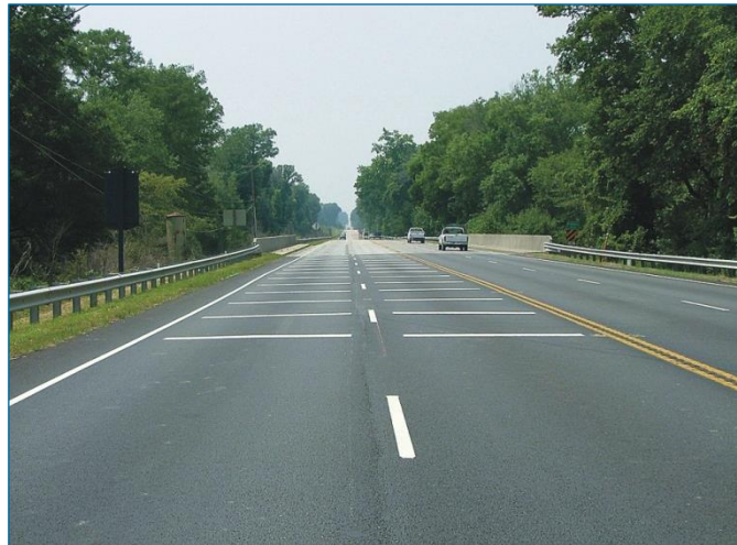
Figure 17. Transverse markings on US 460 (Arnold and Lantz 2007)
