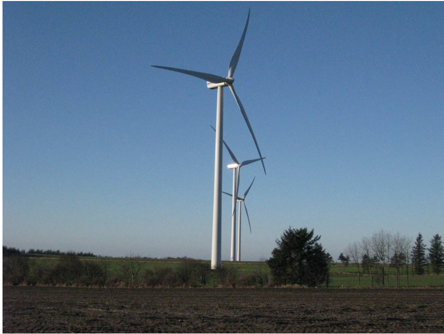
Figure 1.1: Modern upwind, variable-speed, pitch-regulated, horizontal axis wind turbines in operation close to the West coast of Jutland, Denmark.
