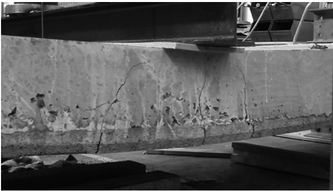
Fig. 6- Ultimate bending failure of a SL-Deck element.
