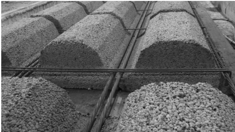
Fig. 2- Casting of SL-deck prototype test elements.
