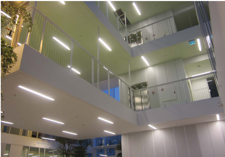
Figure 5.2: View of some of the finished super-light bridge elements.
