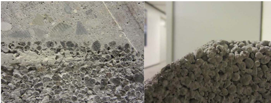
Figure 2.6: On the left cross-section of a fully cast element, on the right comparison with the block without cast concrete.
