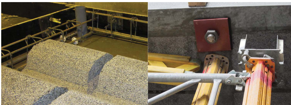
Figure 5.3: Internal beams in the super-light element, on the left before normal concrete is cast on the right how the beams are visible in the final product. The steel parts are interim supports and the nut plate support a hanger carrying the element.
