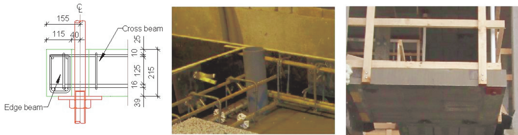
Figure 9: Hanger supports of super-light indoor pedestrian bridge at an element end, on the left production drawing, in the middle setup prior to casting, on the right connection in-situ
