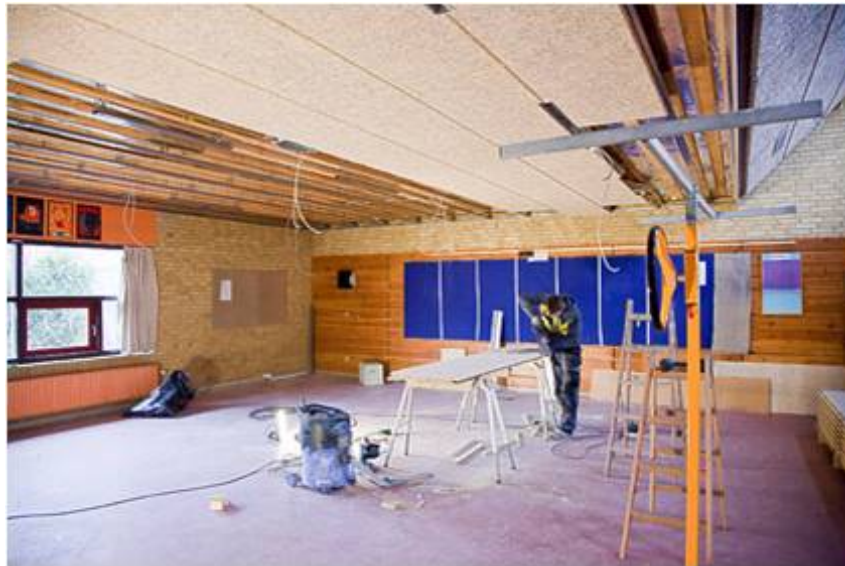
Figure 2. Picture during the installation of the diffuse ventilation inlet.
