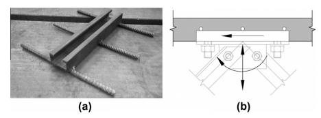
Fig. 9. (a) Cast-in anchor. (b) Resultant forces expected in cast-in anchor, forces shown in vertical and longitudinal direction.
