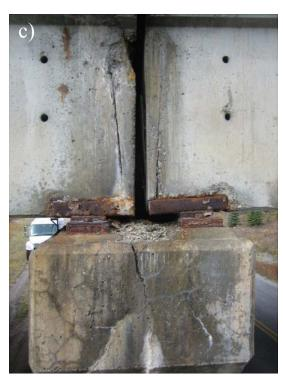
Figure 1-1 Examples of damage due to deterioration of expansion joints, a): in pavement on top of expansion joint (WSDOT, 2011), b): in severely corroded expansion joint seen from below (TCPI, 2012) and c): in girders and pier caps with highly corroded steel bearings (Ho and Lukashnko, 2011).
