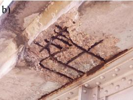
Figure 5-1 Examples of damage due to deterioration and leaching of expansion joints. a): A corroded bridge cantilever pylon below expansion joint and b): a highly corroded R/C deck due to a poorly maintained joint (Webb, 2005).
