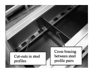
**Fig. 7.** Cut-outs in the steel profiles and cross bracing between steel profile pairs before ECC was cast.
