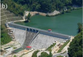
Figure 2-3 Examples of structural applications of SHCC/ECC: a) A continuous steel reinforced ECC link slab in Michigan 2005 (Li and Lepech, 2009). b) The Mitaka Dam on Nishi-Nomi island in Japan, where the up-stream side of the dam was retrofitted with a thin overlay of ECC in 2003 (JDF, 2012).
