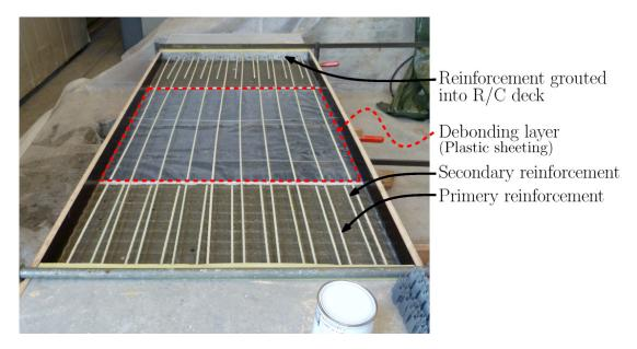
Figure 5-11 Primary and secondary GFRP reinforcement grouted into the R/C deck structure as well as debonding layer centered between the two adjacent deck structures prior to casting LS3 in place.
