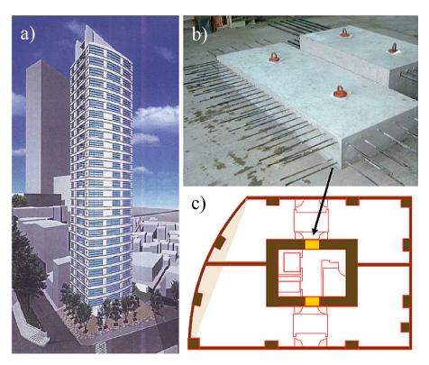
Figure 2-4 Example of ECC used in steel reinforced dampers in high-rise reinforced concrete buildings in Tokyo and Yokohama in 2004 and 2005 (Maruta et al. 2005; Kunieda and Rokugo, 2006).
