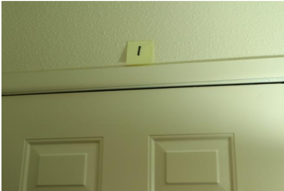
Figure 8 Sticky note marks on the wall after tilt camera
