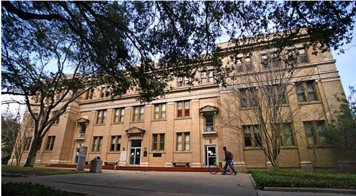
Figure 1 Southwest façade of Francis Hall
